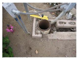
Photograph 10. Suspected ground water supply well.
