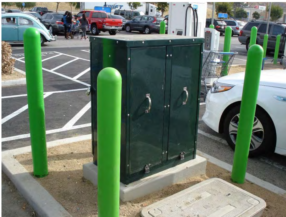
Photo 34 – View of Walmart (4001 Hallmark Parkway) facing northeast. One pad-mounted electrical vehicle distribution unit for electrical vehicles was noted.
