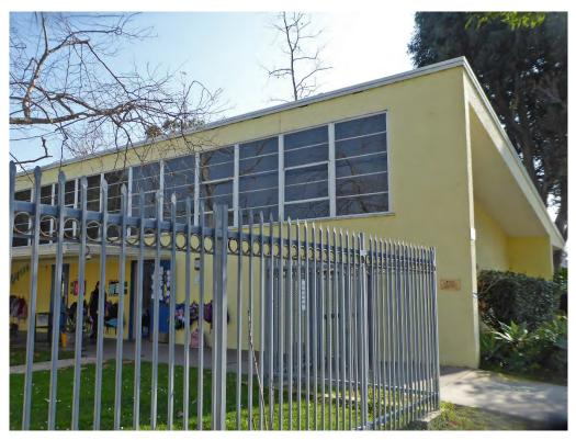
Figure 73. Pacific Elementary School. Detail view of a typical classroom building showing clerestory windows and steep shed roof.
