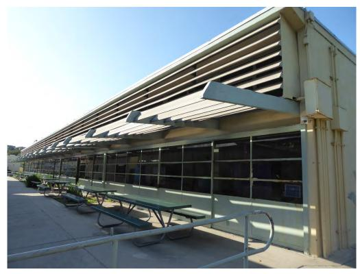
Figure 35. The south façade of Building E, showing metal louvers, pergola, and sliding glass windows and doors.
