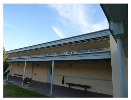
Figure 42. The covered flat canopy and clerestory windows at the north façade of Building G.
