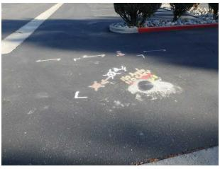
7. View of markings and soil boring from a recent geotechnical investigation
