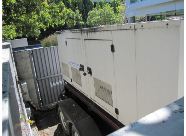
Photograph 8. One of two emergency generators.
