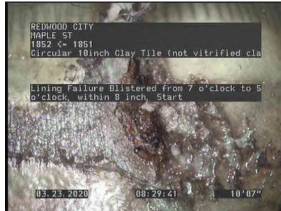
6, 00:02:46, 10.60ft Lining Failure Blistered from 7 o'clock to 5 o'clock, within 8 inch, Start
