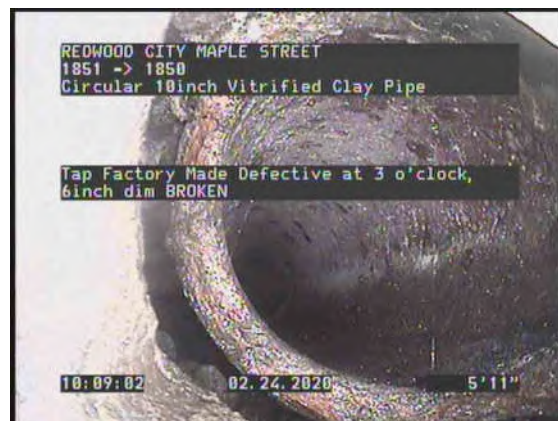
4, 00:01:21, 5.89ft Tap Factory Made Defective at 3 o'clock, 6inch dim / BROKEN
