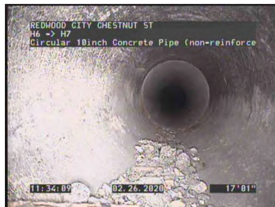
4, 00:01:26, 17.06ft Deposits Attached Grease, 5% of cross sectional area from 5 o'clock to 7 o'clock
