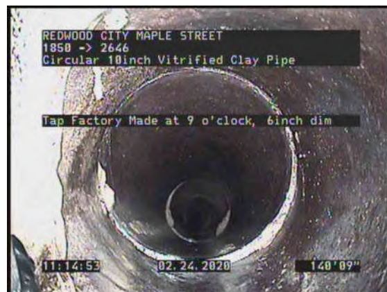
12, 00:08:01, 140.74ft Tap Factory Made at 9 o'clock, 6inch dim
