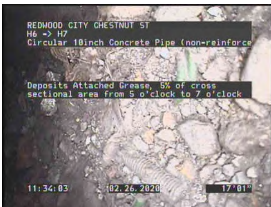
3, 00:01:26, 17.06ft Deposits Attached Grease, 5% of cross sectional area from 5 o'clock to 7 o'clock
