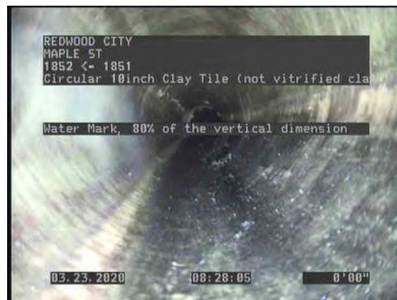
4, 00:01:10, 0.00ft Water Mark, 80% of the vertical dimension
