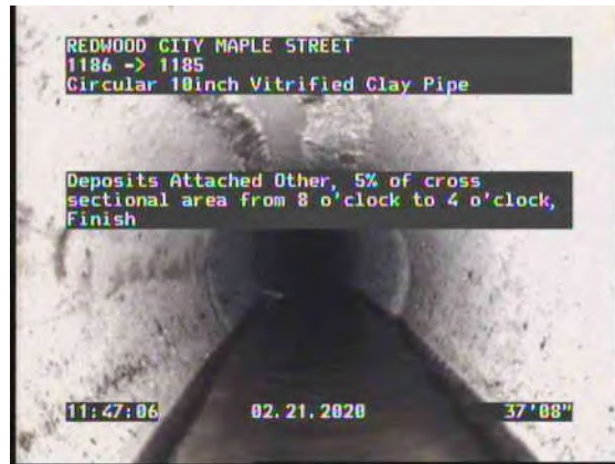
10, 00:05:48, 37.70ft Deposits Attached Other, 5% of cross sectional area from 8 o'clock to 4 o'clock, Finish
