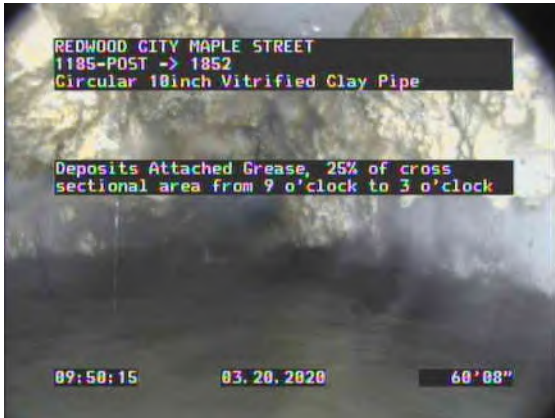
13, 00:11:52, 60.45ft Deposits Attached Grease, 25% of cross sectional area from 9 o'clock to 3 o'clock
