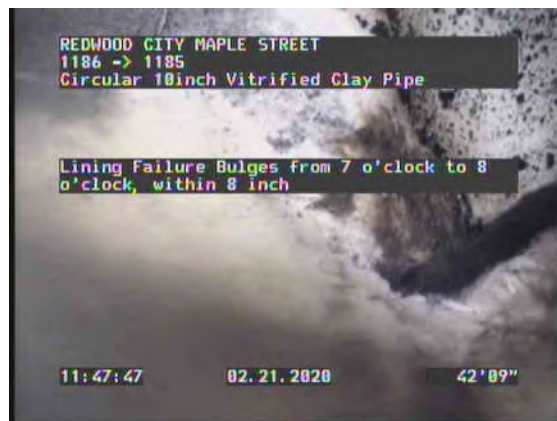
12, 00:06:13, 42.79ft Lining Failure Bulges from 7 o'clock to 8 o'clock, within 8 inch
