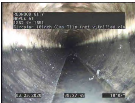
7, 00:02:46, 10.60ft Lining Failure Blistered from 7 o'clock to 5 o'clock, within 8 inch, Start
