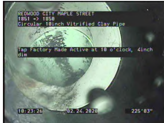
18, 00:14:04, 225.22ft Tap Factory Made Active at 10 o'clock, 4inch dim
