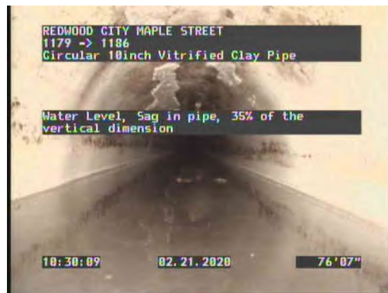
20, 00:08:22, 76.60ft Water Level, Sag in pipe, 35% of the vertical dimension
