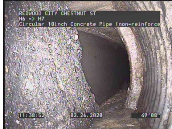
14, 00:05:00, 53.06ft Survey Abandoned / JOINT OFFSET LARGE
