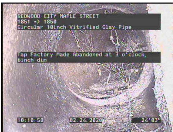
7, 00:02:54, 24.24ft Tap Factory Made Abandoned at 3 o'clock, 6inch dim
