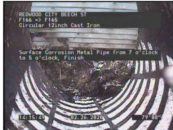
6, 00:03:38, 79.70ft Surface Corrosion Metal Pipe from 7 o'clock to 5 o'clock, Finish
