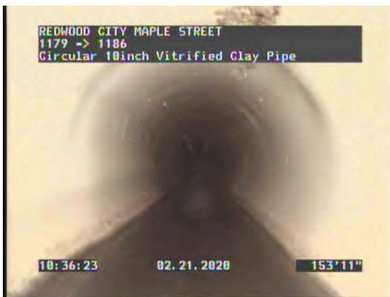
35, 00:13:22, 153.91ft Deposits Attached Grease, 5% of cross sectional area at 1 o'clock
