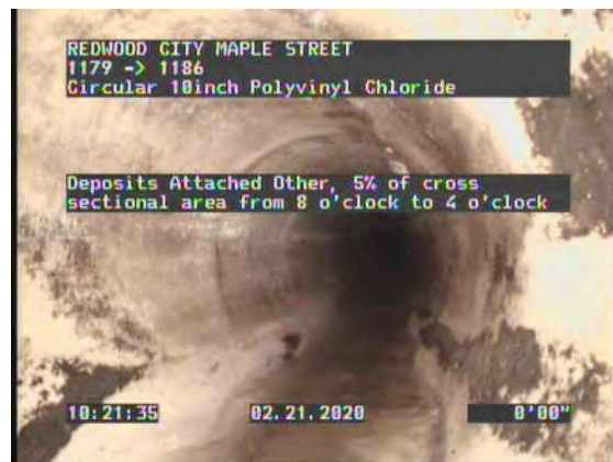
4, 00:00:49, 0.00ft Deposits Attached Other, 5% of cross sectional area from 8 o'clock to 4 o'clock
