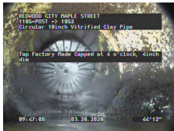
12, 00:08:58, 44.99ft Tap Factory Made Capped at 4 o'clock, 4inch dim
