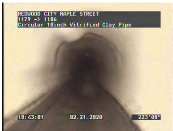
47, 00:18:25, 223.63ft Lining Failure Bulges from 8 o'clock to 4 o'clock, within 8 inch
