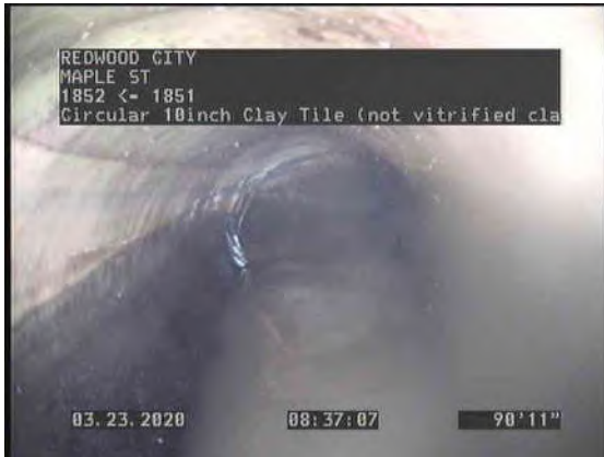
17, 00:09:31, 90.93ft Deposits Attached Grease, 5% of cross sectional area from 11 o'clock to 1 o'clock, within 8 inch, Finish
