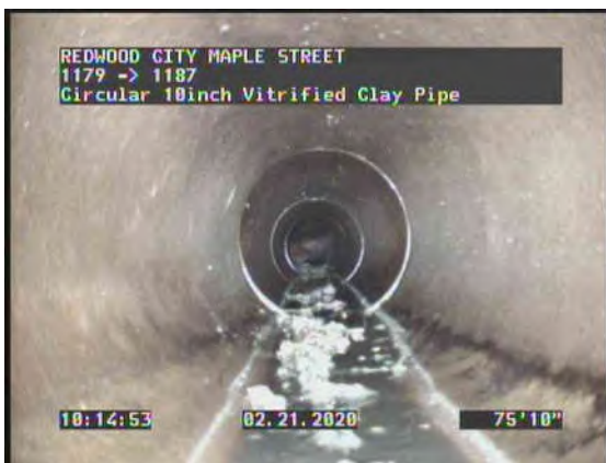
23, 00:07:42, 75.81ft Deposits Settled Fine, 10% of cross sectional area from 5 o'clock to 7 o'clock
