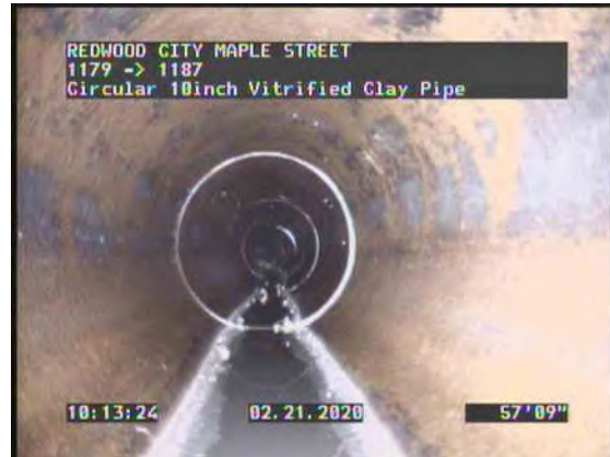
18, 00:06:33, 57.75ft Deposits Attached Grease, 5% of cross sectional area at 10 o'clock, Finish
