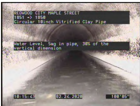
11, 00:07:07, 100.44ft Water Level, Sag in pipe, 30% of the vertical dimension
