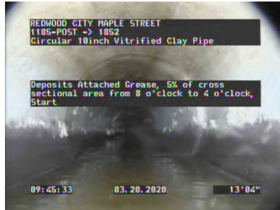
10, 00:07:37, 13.37ft Deposits Attached Grease, 5% of cross sectional area from 8 o'clock to 4 o'clock, Start
