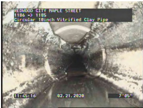
9, 00:04:01, 7.38ft Deposits Attached Grease, 5% of cross sectional area from 10 o'clock to 2 o'clock, Start
