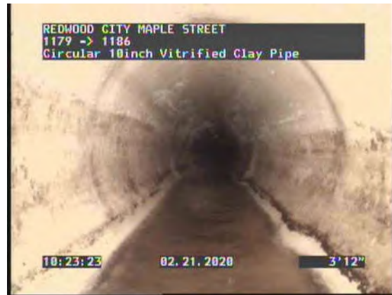
6, 00:02:25, 3.99ft Deposits Attached Other, 5% of cross sectional area from 7 o'clock to 5 o'clock
