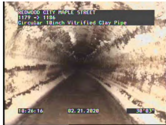
14, 00:04:41, 27.93ft Water Level, Sag in pipe, 20% of the vertical dimension
