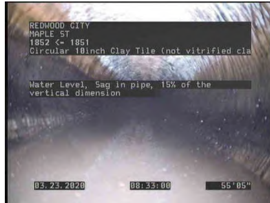
10, 00:06:05, 55.42ft Water Level, Sag in pipe, 15% of the vertical dimension, Start
