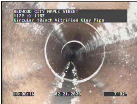
9, 00:02:03, 7.18ft Deposits Attached Grease, 5% of cross sectional area at 2 o'clock, Start
