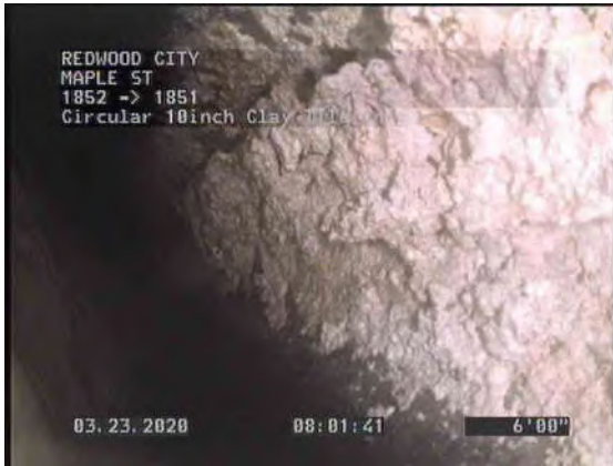
5, 00:01:48, 6.00ft Deposits Attached Grease, 20% of cross sectional area from 10 o'clock to 2 o'clock
