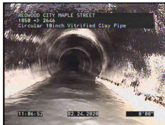
4, 00:00:49, 0.00ft Deposits Attached Other, 5% of cross sectional area from 8 o'clock to 4 o'clock, Start / STAINING
