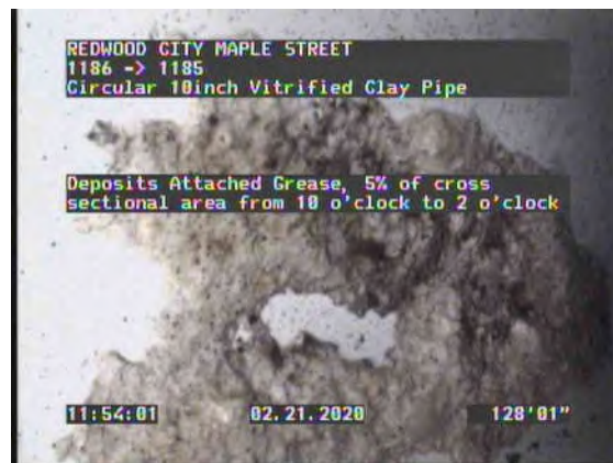
20, 00:11:59, 128.07ft Deposits Attached Grease, 5% of cross sectional area from 10 o'clock to 2 o'clock, Start / WONDERS
