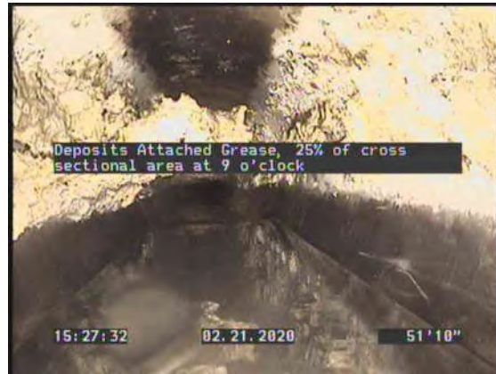
10, 00:03:13, 51.87ft Deposits Attached Grease, 25% of cross sectional area at 9 o'clock
