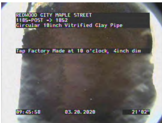
11, 00:07:59, 21.15ft Tap Factory Made at 10 o'clock, 4inch dim
