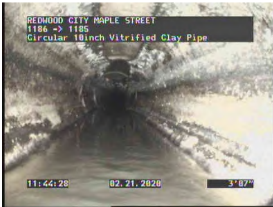
5, 00:03:32, 3.59ft Deposits Attached Grease, 10% of cross sectional area from 10 o'clock to 2 o'clock
