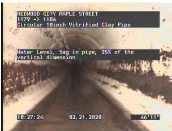
15, 00:05:49, 46.88ft Water Level, Sag in pipe, 25% of the vertical dimension
