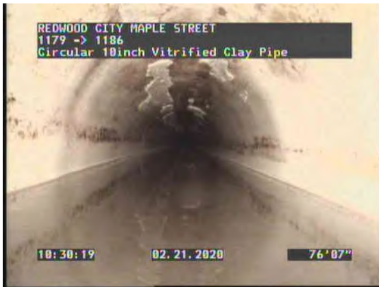
21, 00:08:22, 76.60ft Water Level, Sag in pipe, 35% of the vertical dimension
