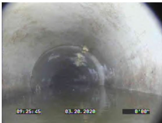
3, 00:00:32, 0.00ft Deposits Attached Other, 5% of cross sectional area from 9 o'clock to 3 o'clock
