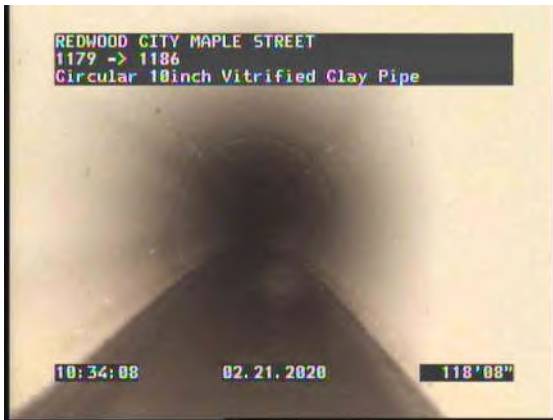
33, 00:11:24, 118.40ft Water Level, Sag in pipe, 25% of the vertical dimension, Start
