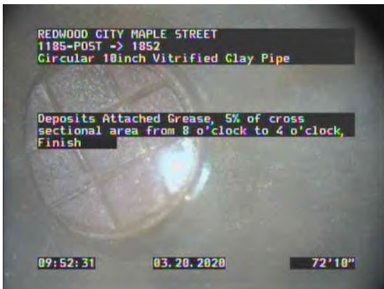
15, 00:13:56, 72.81ft Deposits Attached Grease, 5% of cross sectional area from 8 o'clock to 4 o'clock, Finish
