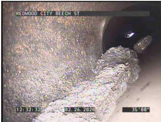
9, 00:02:53, 35.01ft Deposits Settled Fine, 10% of cross sectional area at 8 o'clock
