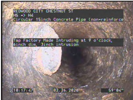
9, 00:04:19, 59.35ft Tap Factory Made Intruding at 9 o'clock, 6inch dim, 3inch intrusion
