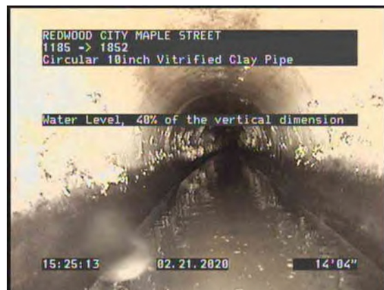
4, 00:01:28, 14.36ft Water Level, 40% of the vertical dimension
