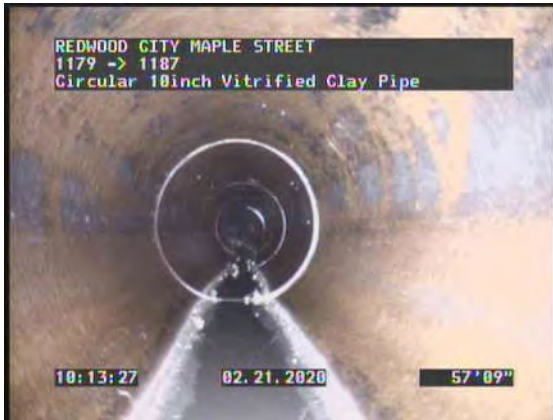
21, 00:06:36, 57.75ft Deposits Attached Grease, 5% of cross sectional area at 2 o'clock, Finish
