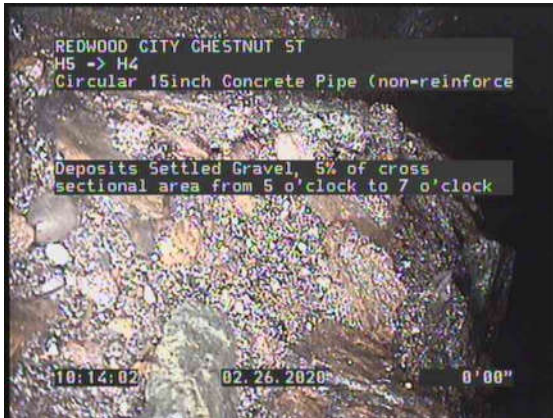
5, 00:01:25, 0.00ft Deposits Settled Gravel, 5% of cross sectional area from 5 o'clock to 7 o'clock
