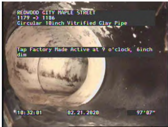
25, 00:09:50, 97.55ft Tap Factory Made Active at 9 o'clock, 6inch dim
