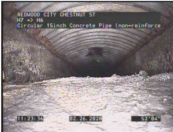
5, 00:03:17, 52.37ft Shape or Size Change, 6inch dim, 8inch dim
