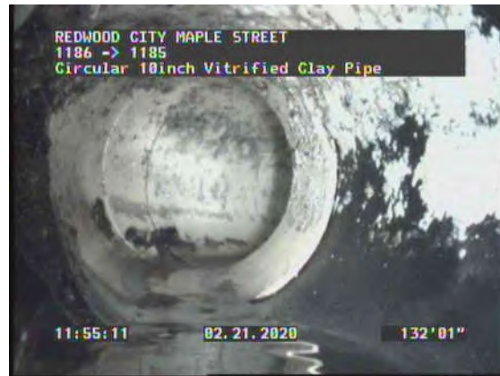
22, 00:12:31, 131.96ft Tap Factory Made at 9 o'clock, 6inch dim
