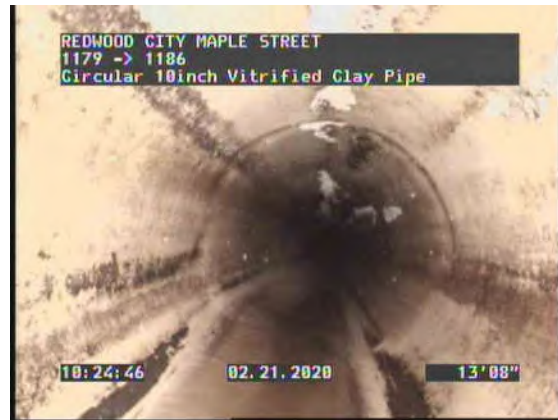
10, 00:03:33, 13.67ft Deposits Attached Other, 5% of cross sectional area from 7 o'clock to 5 o'clock, Start
