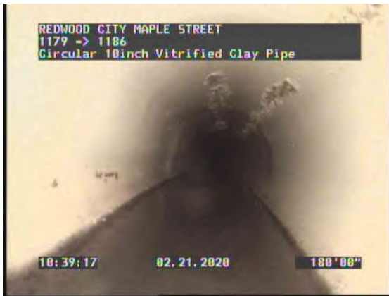
41, 00:15:21, 180.04ft Deposits Attached Grease, 5% of cross sectional area from 11 o'clock to 1 o'clock, Start / DEFECT WONDERS
