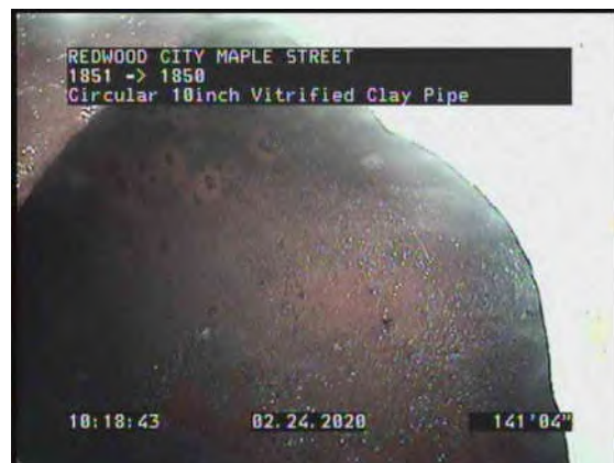
12, 00:09:40, 141.34ft Lining Failure Undercut Connection from 2 o'clock to 5 o'clock
