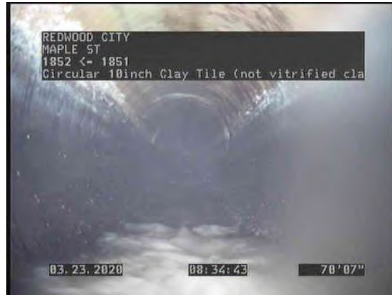
14, 00:07:29, 70.52ft Water Level, Sag in pipe, 15% of the vertical dimension, Finish
