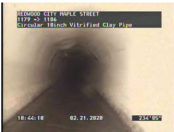
51, 00:19:20, 234.40ft Water Level, Sag in pipe, 25% of the vertical dimension, Start
