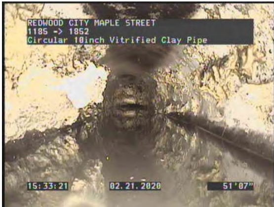
9, 00:06:02, 51.57ft Survey Abandoned / GREASE 50%
