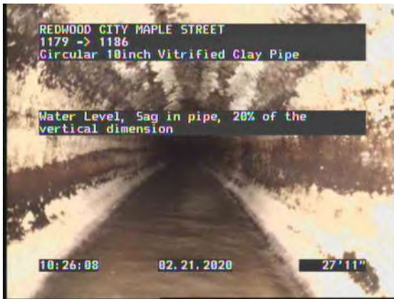
13, 00:04:41, 27.93ft Water Level, Sag in pipe, 20% of the vertical dimension
