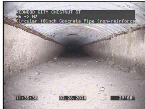
6, 00:02:30, 29.03ft Shape or Size Change, 8inch dim, 10inch dim
