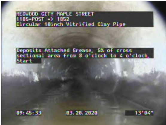
9, 00:07:37, 13.37ft Deposits Attached Grease, 5% of cross sectional area from 8 o'clock to 4 o'clock, Start
