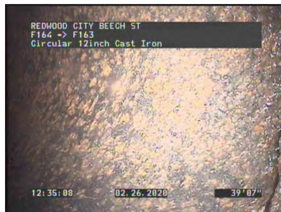
4, 00:03:39, 0.00ft Surface Corrosion Metal Pipe from 8 o'clock to 4 o'clock
