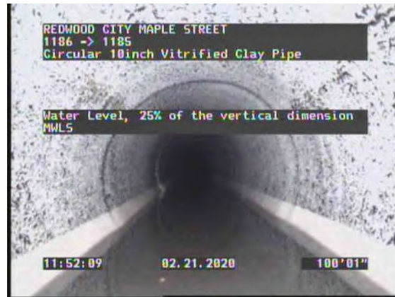
18, 00:09:58, 96.45ft Water Level, 25% of the vertical dimension / MWLS
