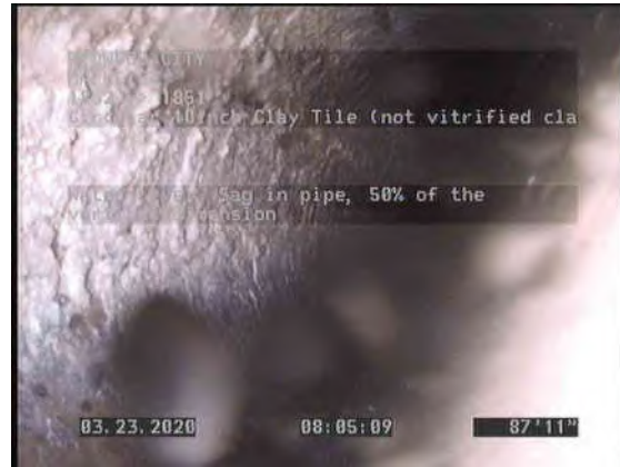
6, 00:05:19, 87.93ft Water Level, Sag in pipe, 50% of the vertical dimension
