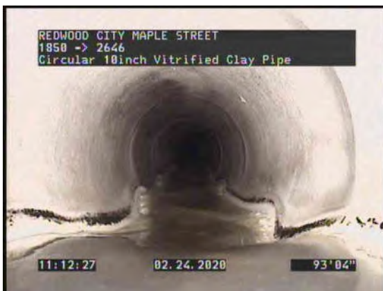
11, 00:05:40, 92.16ft Water Level, Sag in pipe, 30% of the vertical dimension
