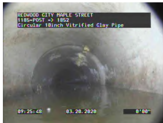
4, 00:00:32, 0.00ft Deposits Attached Other, 5% of cross sectional area from 9 o'clock to 3 o'clock
