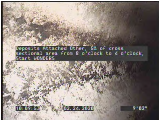
5, 00:02:00, 9.18ft Deposits Attached Other, 5% of cross sectional area from 8 o'clock to 4 o'clock, Start / WONDERS
