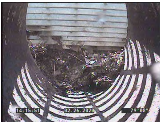
7, 00:03:38, 79.70ft Surface Corrosion Metal Pipe from 7 o'clock to 5 o'clock, Finish
