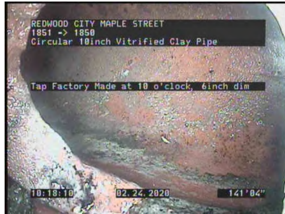
14, 00:09:28, 141.34ft Tap Factory Made Active at 10 o'clock, 6inch dim
