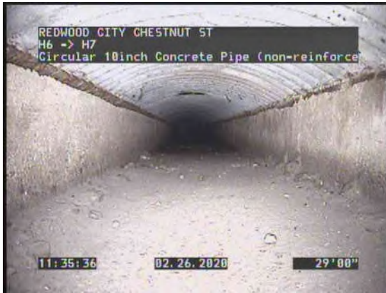
5, 00:02:30, 29.03ft Shape or Size Change, 8inch dim, 10inch dim
