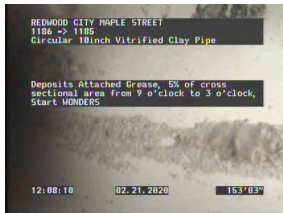
24, 00:17:45, 153.21ft Deposits Attached Grease, 5% of cross sectional area from 8 o'clock to 4 o'clock, Start / WONDERS
