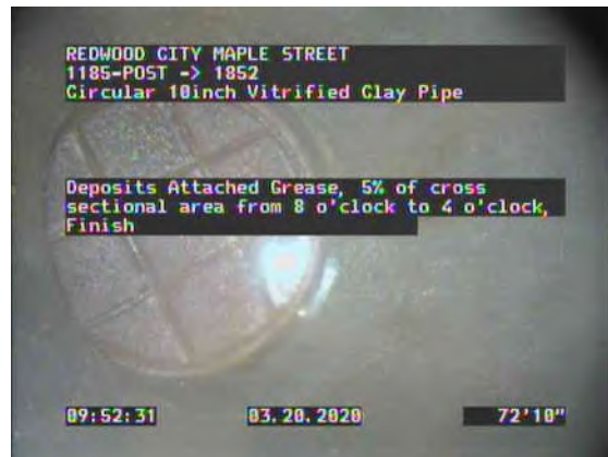
16, 00:13:56, 72.81ft Deposits Attached Grease, 5% of cross sectional area from 8 o'clock to 4 o'clock, Finish
