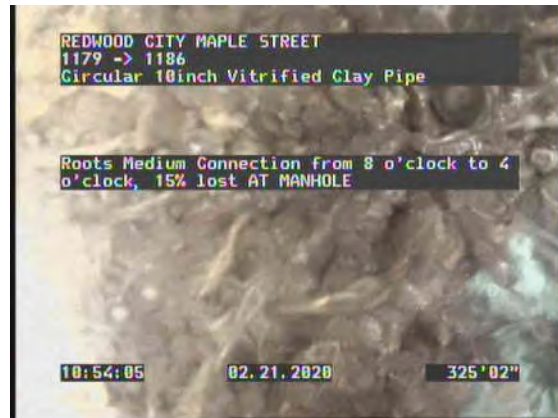
62, 00:26:48, 325.17ft Roots Medium Connection from 8 o'clock to 4 o'clock, 15% lost / AT MANHOLE
