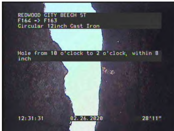
5, 00:02:10, 28.93ft Hole from 10 o'clock to 2 o'clock, within 8 inch
