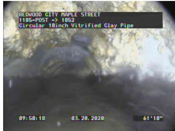
14, 00:11:52, 60.45ft Deposits Attached Grease, 25% of cross sectional area from 9 o'clock to 3 o'clock
