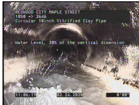
2, 00:00:46, 0.00ft Water Level, 20% of the vertical dimension
