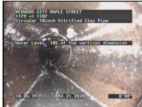
2, 00:00:39, 0.00ft Water Level, 10% of the vertical dimension
