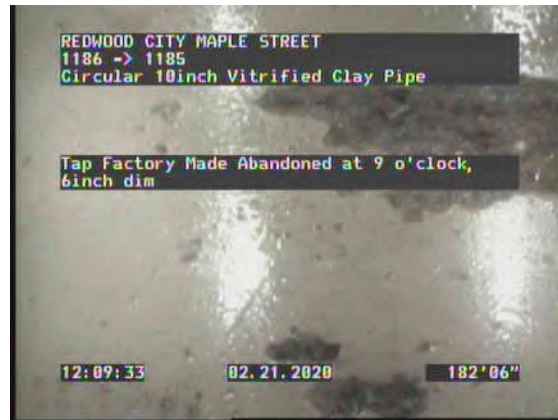
26, 00:18:54, 182.53ft Tap Factory Made Abandoned at 9 o'clock, 6inch dim
