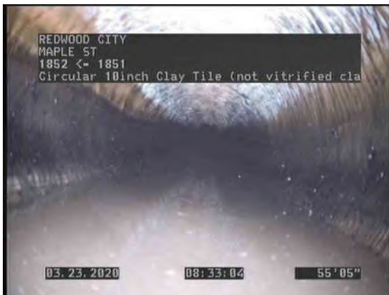
11, 00:06:05, 55.42ft Water Level, Sag in pipe, 15% of the vertical dimension, Start
