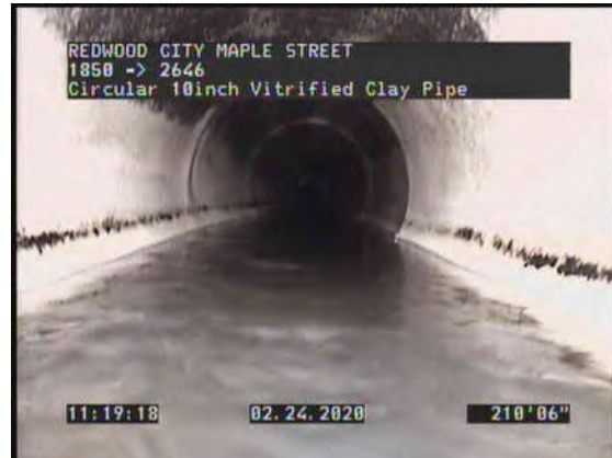
14, 00:12:13, 209.66ft Water Level, Sag in pipe, 35% of the vertical dimension, Start
