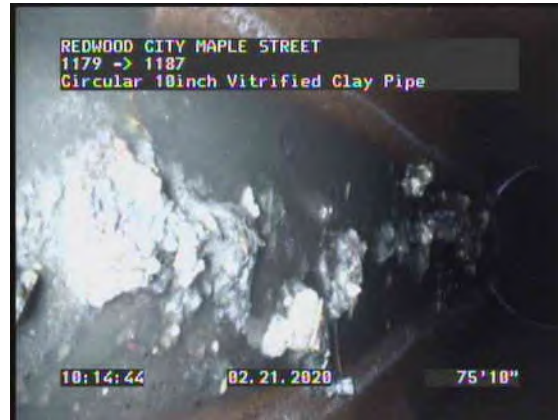
22, 00:07:42, 75.81ft Deposits Settled Fine, 10% of cross sectional area from 5 o'clock to 7 o'clock
