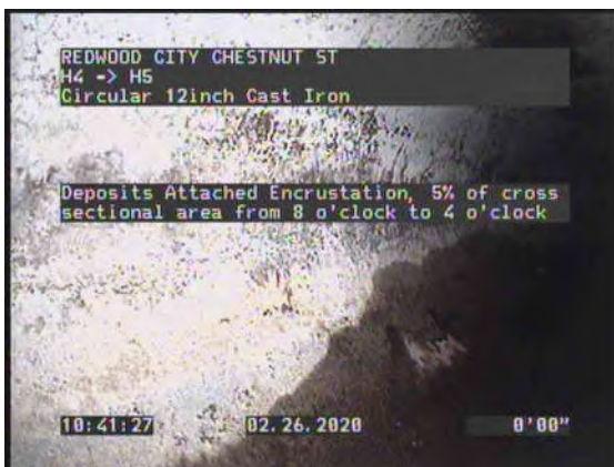
3, 00:01:06, 0.00ft Deposits Attached Encrustation, 5% of cross sectional area from 8 o'clock to 4 o'clock
