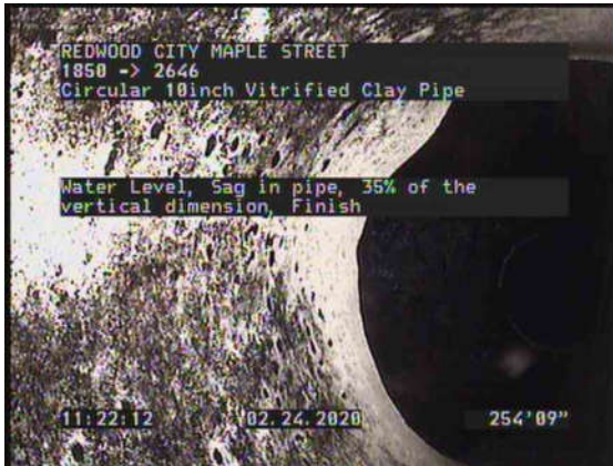
17, 00:14:59, 254.75ft Water Level, Sag in pipe, 35% of the vertical dimension, Finish
