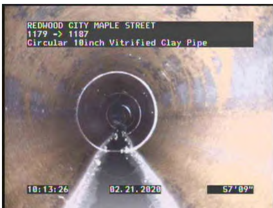
19, 00:06:33, 57.75ft Deposits Attached Grease, 5% of cross sectional area at 10 o'clock, Finish
