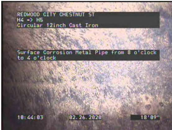
9, 00:03:14, 18.75ft Surface Corrosion Metal Pipe from 8 o'clock to 4 o'clock
