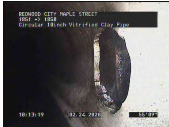
10, 00:04:42, 55.76ft Lining Failure Overcut Connection from 7 o'clock to 10 o'clock
