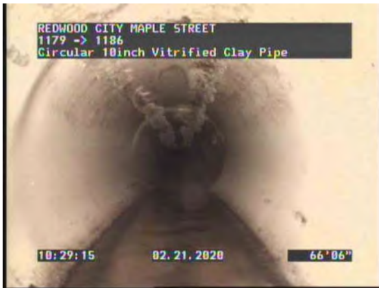
17, 00:07:34, 66.53ft Deposits Attached Other, 5% of cross sectional area from 7 o'clock to 5 o'clock, Finish
