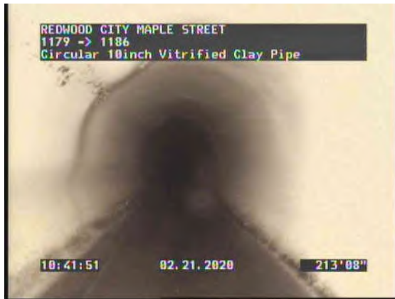
45, 00:17:25, 213.65ft Lining Failure Bulges from 8 o'clock to 4 o'clock, within 8 inch
