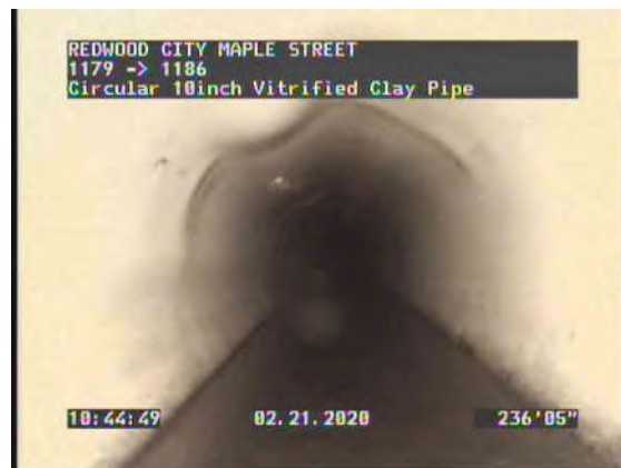
52, 00:19:45, 236.40ft Lining Failure Bulges from 9 o'clock to 3 o'clock
