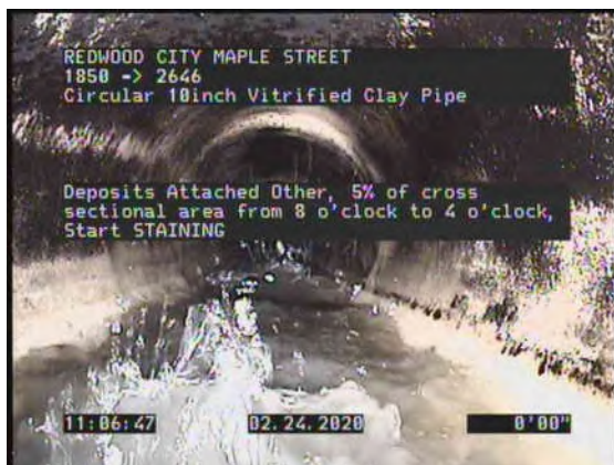
3, 00:00:49, 0.00ft Deposits Attached Other, 5% of cross sectional area from 8 o'clock to 4 o'clock, Start / STAINING
