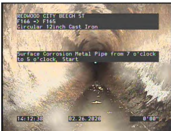
3, 00:00:37, 0.00ft Surface Corrosion Metal Pipe from 7 o'clock to 5 o'clock, Start
