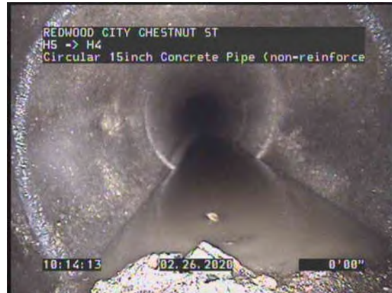
6, 00:01:25, 0.00ft Deposits Settled Gravel, 5% of cross sectional area from 5 o'clock to 7 o'clock
