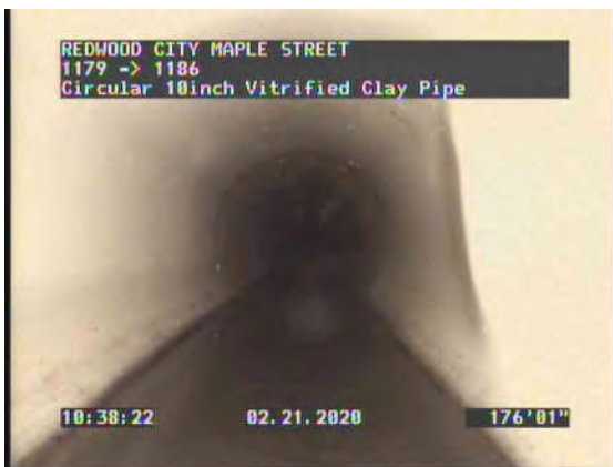
39, 00:14:52, 176.05ft Lining Failure Bulges at 3 o'clock
