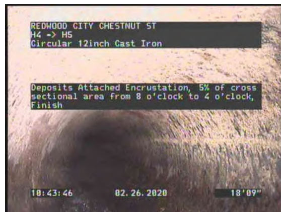
8, 00:03:06, 18.75ft Deposits Attached Encrustation, 5% of cross sectional area from 8 o'clock to 4 o'clock, Finish
