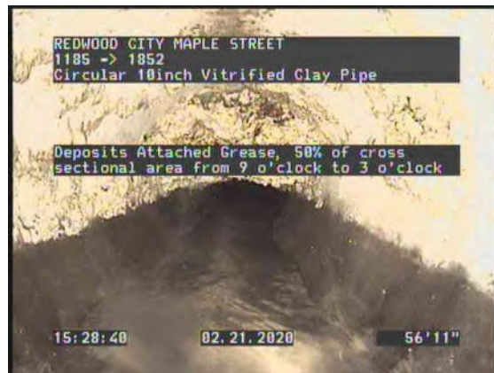
12, 00:04:14, 56.95ft Deposits Attached Grease, 50% of cross sectional area from 9 o'clock to 3 o'clock
