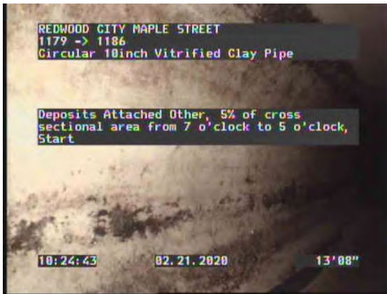
9, 00:03:33, 13.67ft Deposits Attached Other, 5% of cross sectional area from 7 o'clock to 5 o'clock, Start
