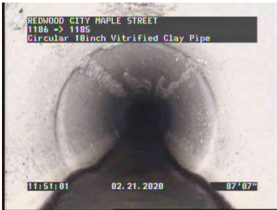
17, 00:09:10, 87.58ft Deposits Attached Grease, 5% of cross sectional area from 10 o'clock to 2 o'clock
