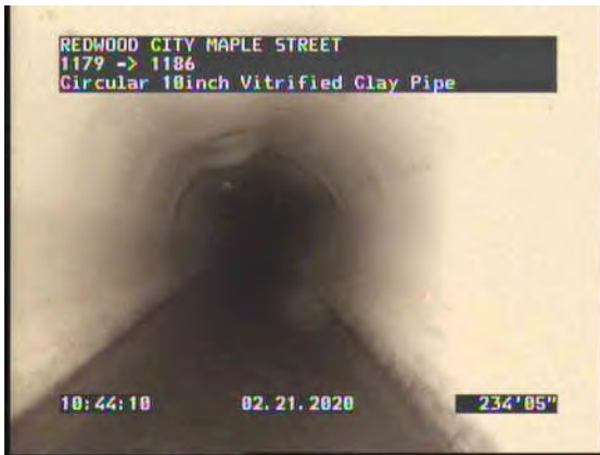
49, 00:18:58, 228.22ft Water Level, Sag in pipe, 25% of the vertical dimension, Finish
