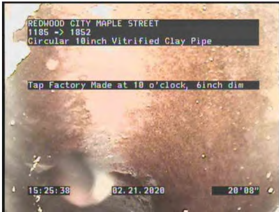
5, 00:01:45, 20.65ft Tap Factory Made at 10 o'clock, 6inch dim
