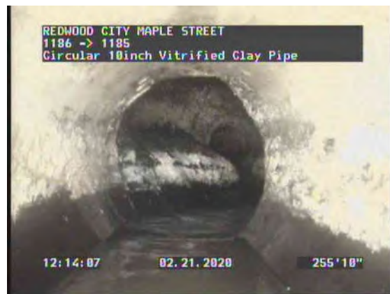
32, 00:22:45, 255.75ft Deposits Attached Grease, 5% of cross sectional area from 8 o'clock to 4 o'clock, Finish / WONDERS
