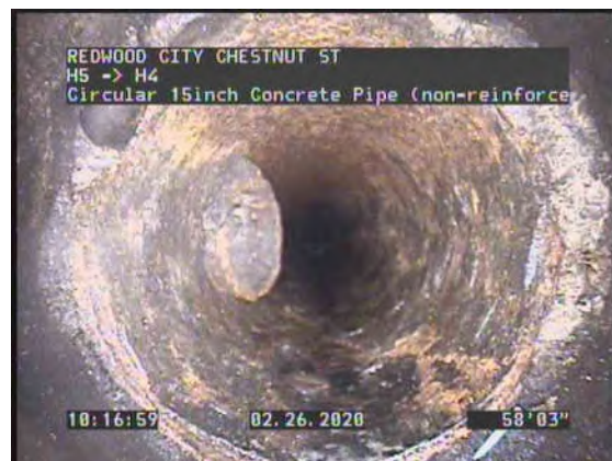
8, 00:03:50, 58.25ft Material Change, Cast iron / CP TO CAST IRON 12 INCH
