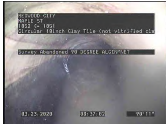
18, 00:09:53, 90.93ft Survey Abandoned / 90 DEGREE ALGINMNET
