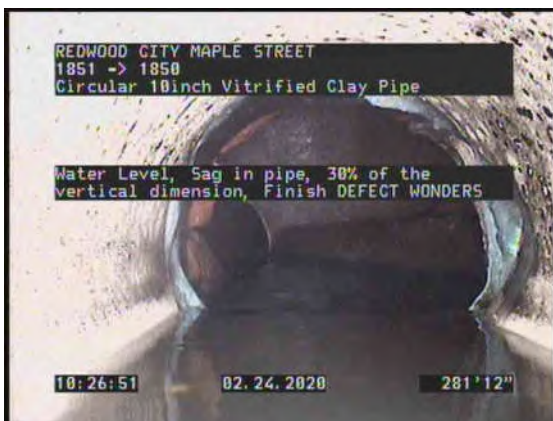
19, 00:17:25, 281.98ft Water Level, Sag in pipe, 30% of the vertical dimension, Finish / DEFECT WONDERS
