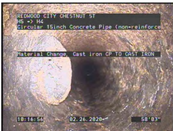
7, 00:03:50, 58.25ft Material Change, Cast iron / CP TO CAST IRON 12 INCH
