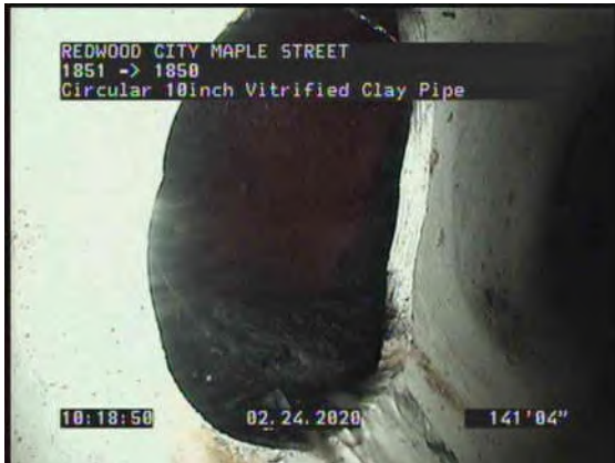
13, 00:09:40, 141.34ft Lining Failure Undercut Connection from 2 o'clock to 5 o'clock
