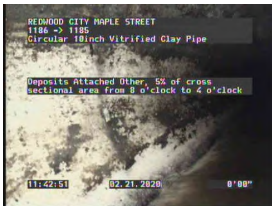
3, 00:02:11, 0.00ft Deposits Attached Other, 5% of cross sectional area from 8 o'clock to 4 o'clock
