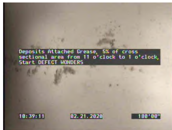
40, 00:15:21, 180.04ft Deposits Attached Grease, 5% of cross sectional area from 11 o'clock to 1 o'clock, Start / DEFECT WONDERS
