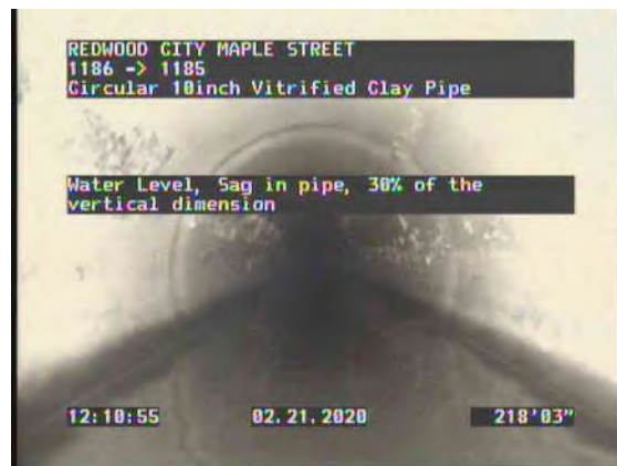
28, 00:20:11, 216.65ft Water Level, Sag in pipe, 30% of the vertical dimension
