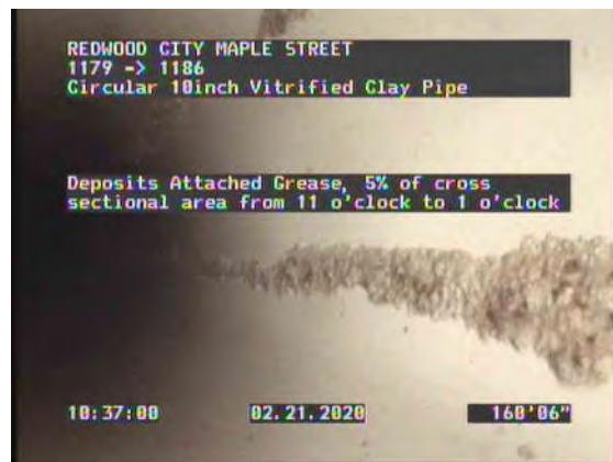
36, 00:14:00, 160.49ft Deposits Attached Grease, 5% of cross sectional area from 11 o'clock to 1 o'clock
