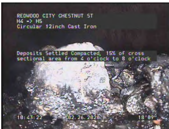
7, 00:02:45, 18.75ft Deposits Settled Compacted, 15% of cross sectional area from 4 o'clock to 8 o'clock
