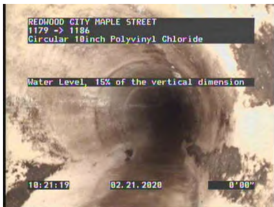
3, 00:00:45, 0.00ft Water Level, 15% of the vertical dimension
