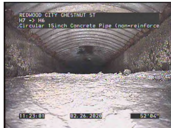
4, 00:03:17, 52.37ft Shape or Size Change, 6inch dim, 8inch dim
