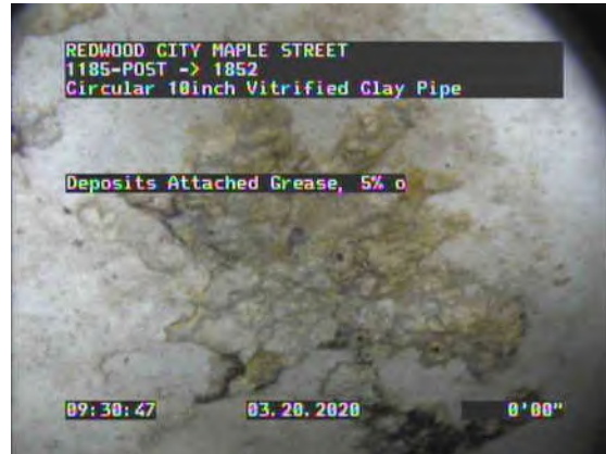
6, 00:05:17, 0.00ft Deposits Attached Grease, 5% of cross sectional area from 11 o'clock to 12 o'clock
