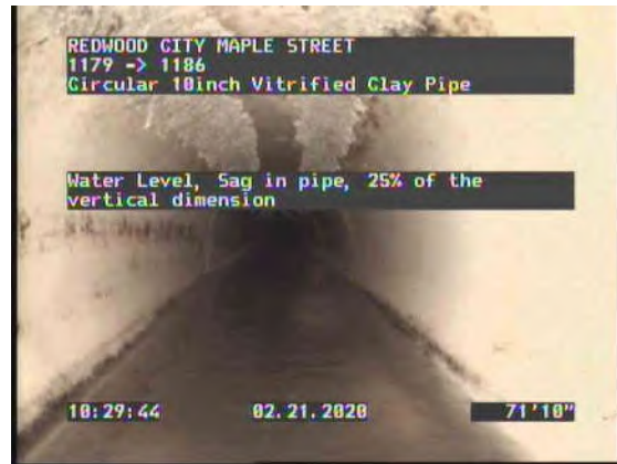
18, 00:07:59, 71.82ft Water Level, Sag in pipe, 25% of the vertical dimension
