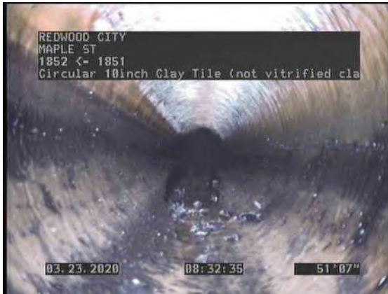
9, 00:05:36, 51.52ft Lining Failure Blistered from 7 o'clock to 5 o'clock, within 8 inch, Finish
