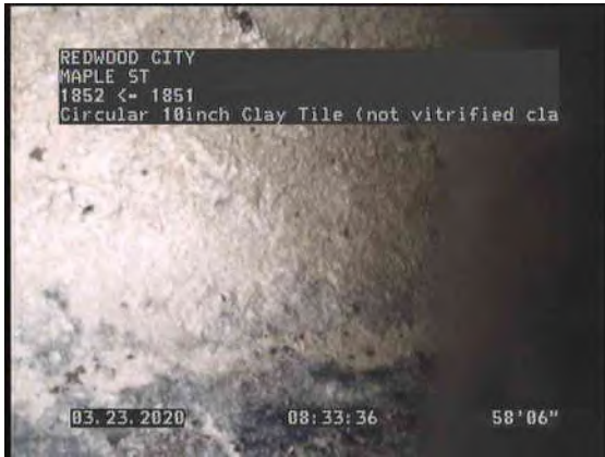
13, 00:06:35, 58.52ft Deposits Attached Grease, 5% of cross sectional area from 11 o'clock to 1 o'clock, within 8 inch, Start
