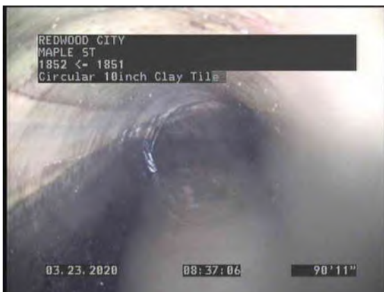
19, 00:09:53, 90.93ft Survey Abandoned / 90 DEGREE ALGINMNET
