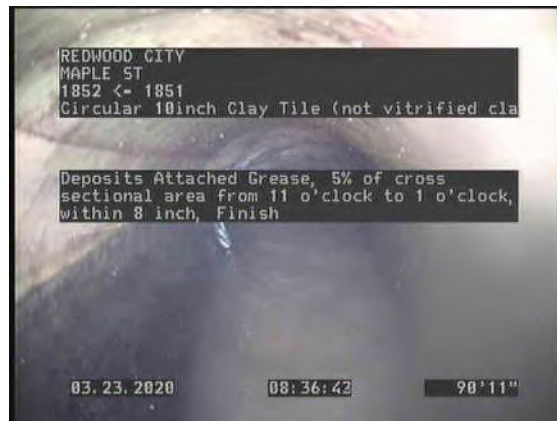
16, 00:09:31, 90.93ft Deposits Attached Grease, 5% of cross sectional area from 11 o'clock to 1 o'clock, within 8 inch, Finish
