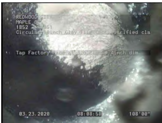
7, 00:06:45, 108.04ft Tap Factory Made at 3 o'clock, 6inch dim
