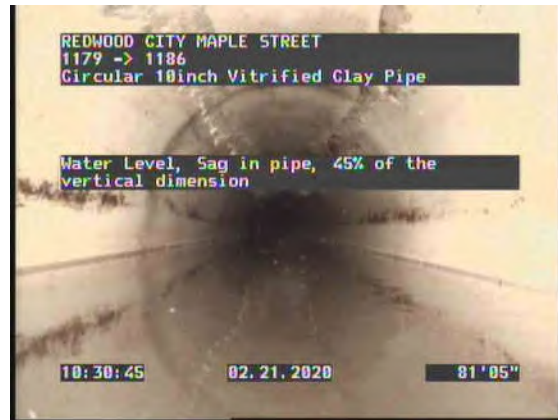
22, 00:08:52, 81.39ft Water Level, Sag in pipe, 45% of the vertical dimension
