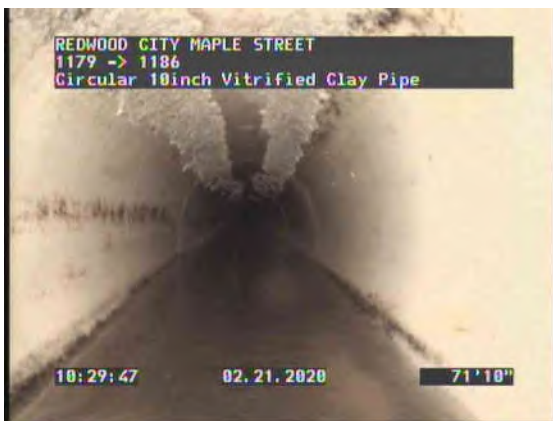
19, 00:07:59, 71.82ft Water Level, Sag in pipe, 25% of the vertical dimension
