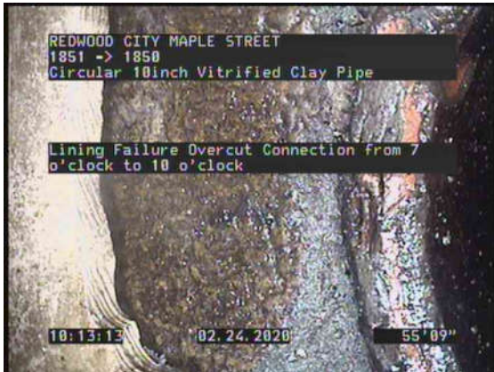
9, 00:04:42, 55.76ft Lining Failure Overcut Connection from 7 o'clock to 10 o'clock
