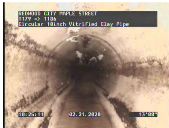
12, 00:03:43, 13.67ft Deposits Attached Grease, 5% of cross sectional area from 11 o'clock to 1 o'clock, Start / WONDERS
