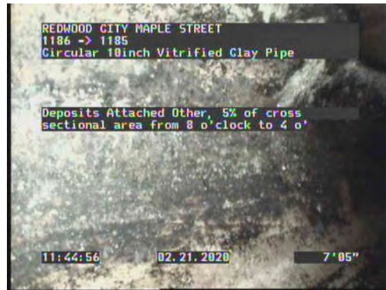
6, 00:03:59, 7.38ft Deposits Attached Other, 5% of cross sectional area from 8 o'clock to 4 o'clock, Start
