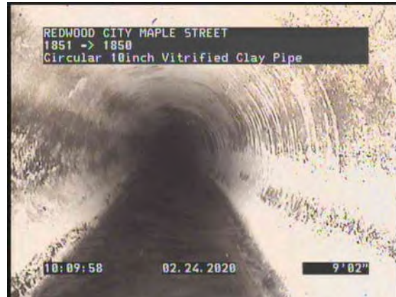
6, 00:02:00, 9.18ft Deposits Attached Other, 5% of cross sectional area from 8 o'clock to 4 o'clock, Start / WONDERS
