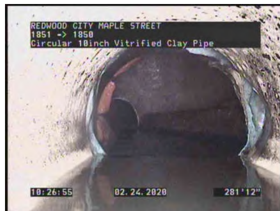
20, 00:17:25, 281.98ft Water Level, Sag in pipe, 30% of the vertical dimension, Finish / DEFECT WONDERS
