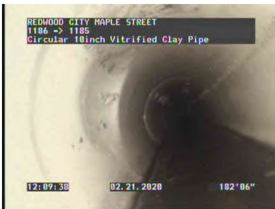
27, 00:18:54, 182.53ft Tap Factory Made Abandoned at 10 o'clock, 6inch dim
