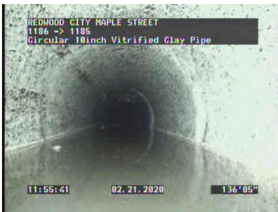
23, 00:13:19, 136.45ft Water Level, 35% of the vertical dimension
