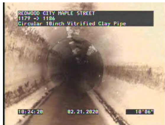
8, 00:03:05, 10.47ft Deposits Attached Grease, 5% of cross sectional area at 11 o'clock
