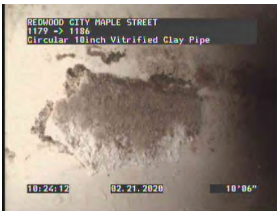
7, 00:03:05, 10.47ft Deposits Attached Grease, 5% of cross sectional area at 11 o'clock
