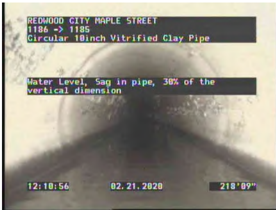
29, 00:20:11, 216.65ft Water Level, Sag in pipe, 30% of the vertical dimension
