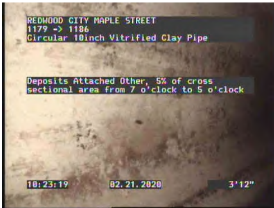
5, 00:02:25, 3.99ft Deposits Attached Other, 5% of cross sectional area from 7 o'clock to 5 o'clock
