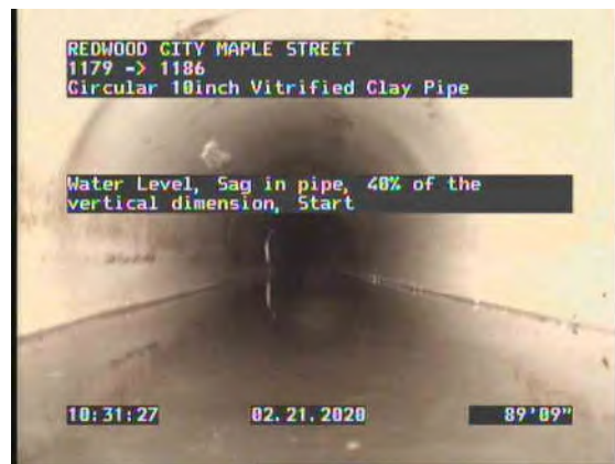
24, 00:09:24, 89.67ft Water Level, Sag in pipe, 40% of the vertical dimension, Start
