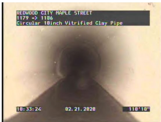
31, 00:10:53, 110.82ft Water Level, Sag in pipe, 25% of the vertical dimension
