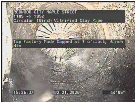
7, 00:02:40, 44.39ft Tap Factory Made Capped at 9 o'clock, 6inch dim
