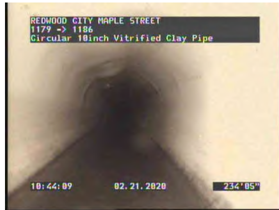
50, 00:19:20, 234.40ft Water Level, Sag in pipe, 25% of the vertical dimension, Start
