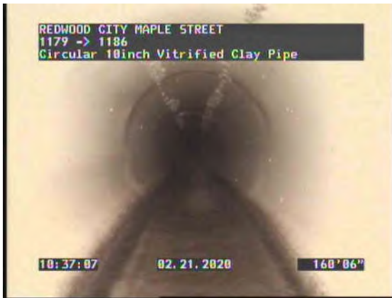
37, 00:14:00, 160.49ft Deposits Attached Grease, 5% of cross sectional area from 11 o'clock to 1 o'clock
