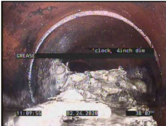
9, 00:03:02, 38.60ft Tap Factory Made at 10 o'clock, 4inch dim / GREASE
