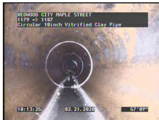
20, 00:06:36, 57.75ft Deposits Attached Grease, 5% of cross sectional area at 2 o'clock, Finish
