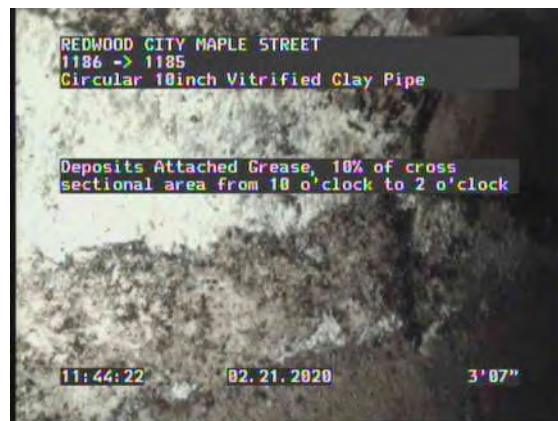
4, 00:03:32, 3.59ft Deposits Attached Grease, 10% of cross sectional area from 10 o'clock to 2 o'clock
