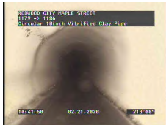
44, 00:17:25, 213.65ft Lining Failure Bulges from 8 o'clock to 4 o'clock, within 8 inch
