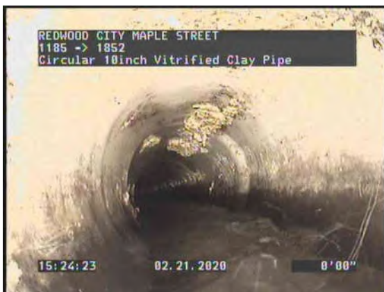
3, 00:00:38, 0.00ft Deposits Attached Grease, 10% of cross sectional area from 8 o'clock to 4 o'clock / DEFECT WONDERS
