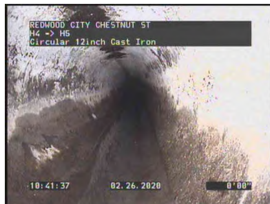
4, 00:01:06, 0.00ft Deposits Attached Encrustation, 5% of cross sectional area from 8 o'clock to 4 o'clock
