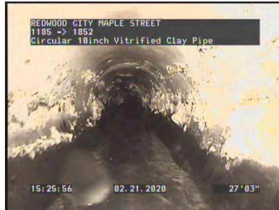
6, 00:01:45, 20.65ft Tap Factory Made at 10 o'clock, 6inch dim
