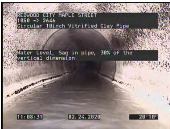
7, 00:02:07, 20.85ft Water Level, Sag in pipe, 30% of the vertical dimension
