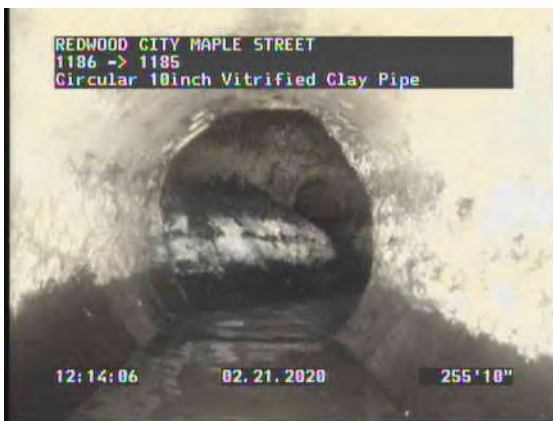
31, 00:22:45, 255.75ft Deposits Attached Grease, 5% of cross sectional area from 8 o'clock to 4 o'clock, Finish / WONDERS
