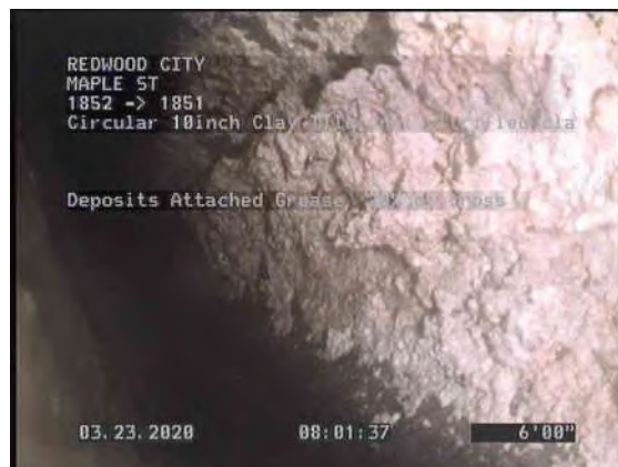
4, 00:01:48, 6.00ft Deposits Attached Grease, 20% of cross sectional area from 10 o'clock to 2 o'clock
