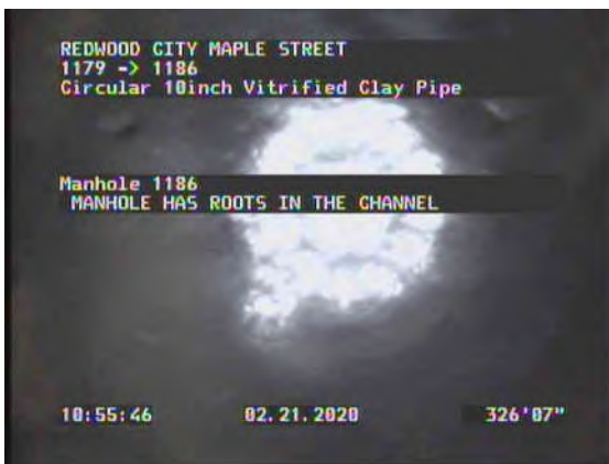
63, 00:27:13, 326.57ft Manhole / 1186 MANHOLE HAS ROOTS IN THE CHANNEL
