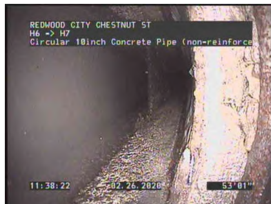
12, 00:04:43, 53.06ft Joint Offset Large, 1Inch
