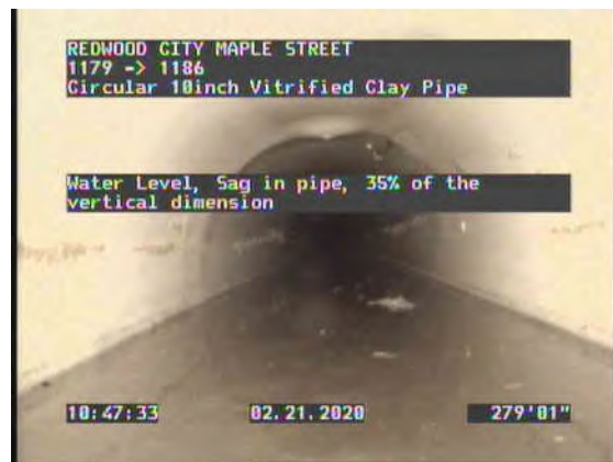
56, 00:22:16, 279.09ft Water Level, Sag in pipe, 35% of the vertical dimension, Start
