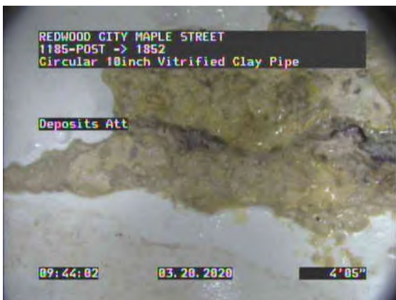
7, 00:06:17, 4.39ft Deposits Attached Grease, 5% of cross sectional area at 2 o'clock
