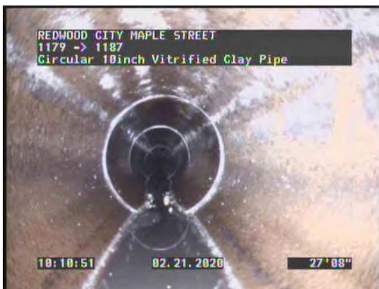
11, 00:03:44, 16.36ft Water Level, Sag in pipe, 15% of the vertical dimension
