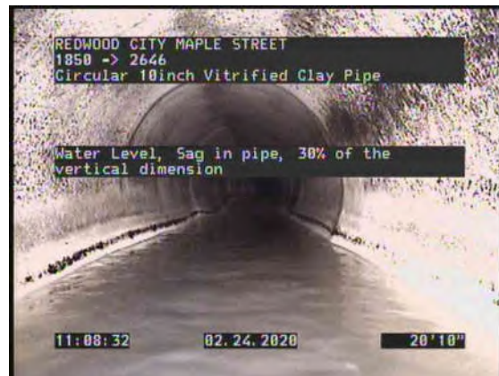
8, 00:02:07, 20.85ft Water Level, Sag in pipe, 30% of the vertical dimension
