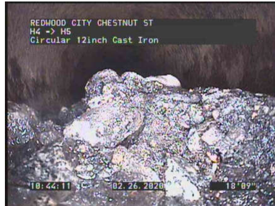
10, 00:03:14, 18.75ft Surface Corrosion Metal Pipe from 8 o'clock to 4 o'clock
