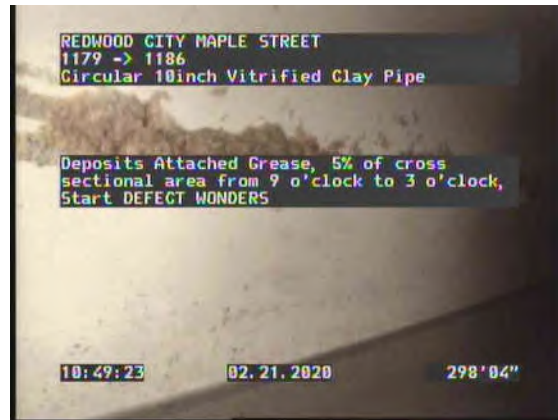
58, 00:23:33, 298.34ft Deposits Attached Grease, 5% of cross sectional area from 9 o'clock to 3 o'clock, Start / DEFECT WONDERS
