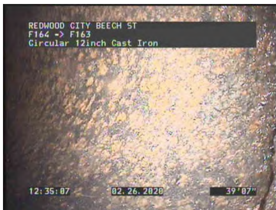
3, 00:03:39, 0.00ft Surface Corrosion Metal Pipe from 8 o'clock to 4 o'clock
