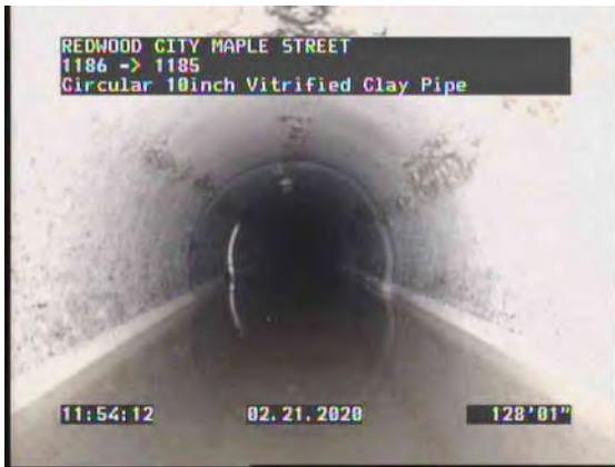
21, 00:11:59, 128.07ft Deposits Attached Grease, 5% of cross sectional area from 10 o'clock to 2 o'clock, Start / WONDERS
