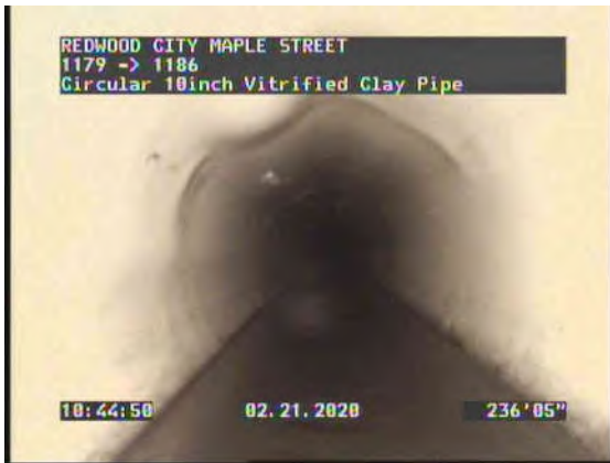
53, 00:19:45, 236.40ft Lining Failure Bulges from 9 o'clock to 3 o'clock
