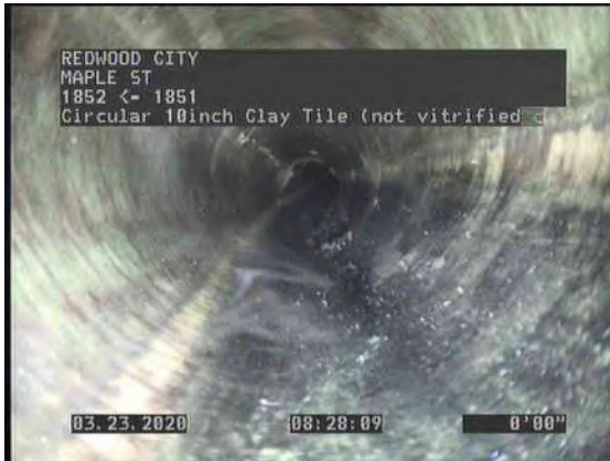
5, 00:01:10, 0.00ft Water Mark, 80% of the vertical dimension
