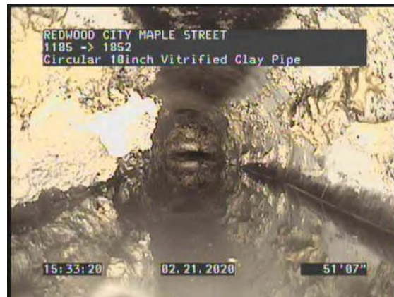
8, 00:06:02, 51.57ft Survey Abandoned / GREASE 50%
