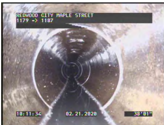
15, 00:05:13, 38.10ft Water Level, Sag in pipe, 15% of the vertical dimension
