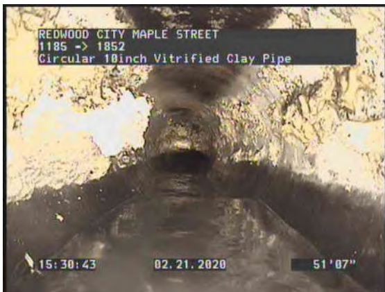
11, 00:03:13, 51.87ft Deposits Attached Grease, 25% of cross sectional area at 9 o'clock
