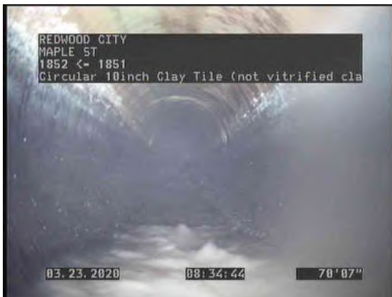
15, 00:07:29, 70.52ft Water Level, Sag in pipe, 15% of the vertical dimension, Finish
