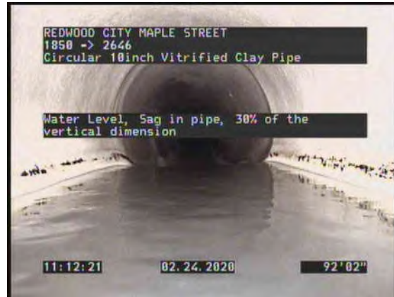
10, 00:05:40, 92.16ft Water Level, Sag in pipe, 30% of the vertical dimension
