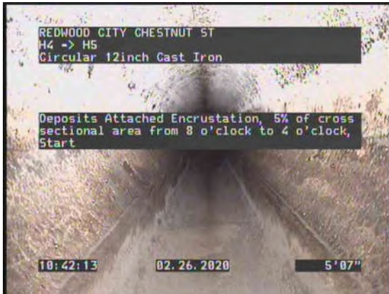
5, 00:01:36, 5.59ft Deposits Attached Encrustation, 5% of cross sectional area from 8 o'clock to 4 o'clock, Start
