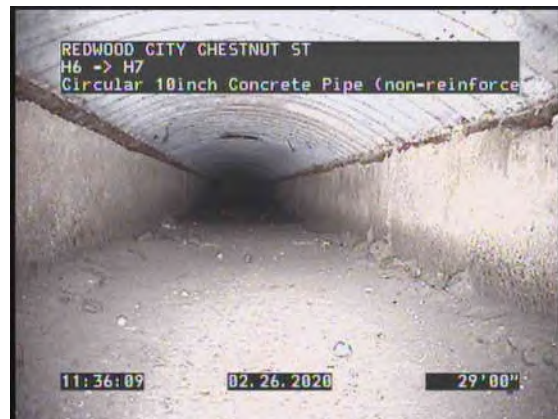
8, 00:02:51, 29.03ft Material Change, Corrugated metal pipe / TOP OF PIPE
