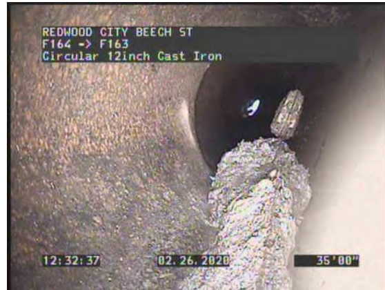
10, 00:02:53, 35.01ft Deposits Settled Fine, 10% of cross sectional area at 8 o'clock
