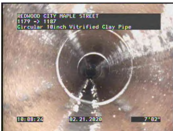
7, 00:01:59, 7.18ft Deposits Attached Grease, 5% of cross sectional area at 10 o'clock, Start
