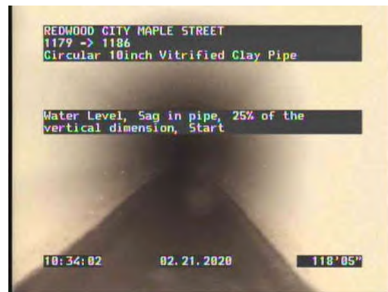
32, 00:11:24, 118.40ft Water Level, Sag in pipe, 25% of the vertical dimension, Start
