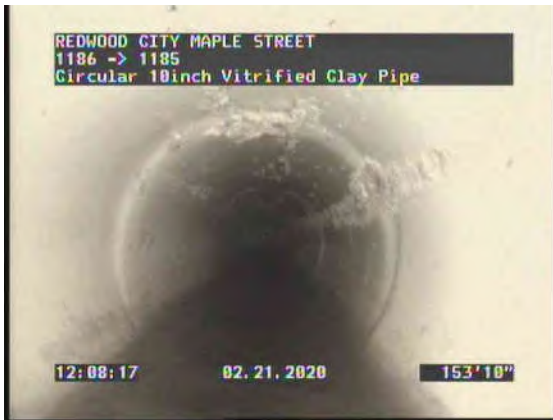
25, 00:17:45, 153.21ft Deposits Attached Grease, 5% of cross sectional area from 8 o'clock to 4 o'clock, Start / WONDERS
