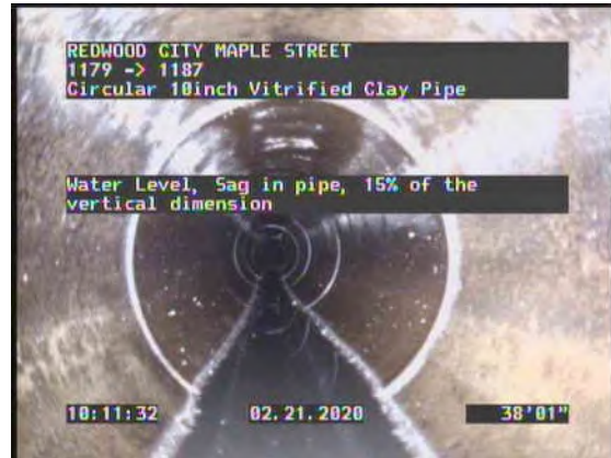
14, 00:05:13, 38.10ft Water Level, Sag in pipe, 15% of the vertical dimension
