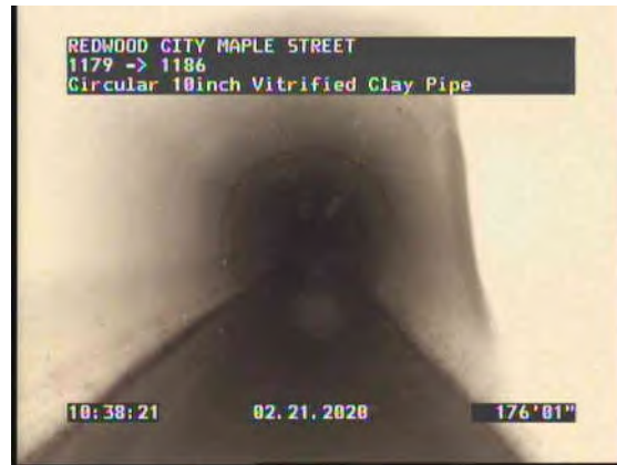
38, 00:14:52, 176.05ft Lining Failure Bulges at 3 o'clock
