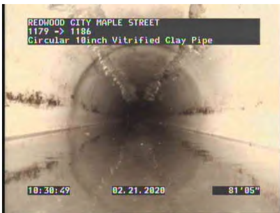
23, 00:08:52, 81.39ft Water Level, Sag in pipe, 45% of the vertical dimension
