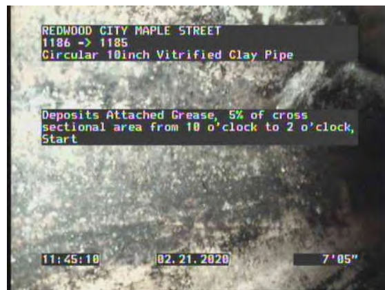
8, 00:04:01, 7.38ft Deposits Attached Grease, 5% of cross sectional area from 10 o'clock to 2 o'clock, Start
