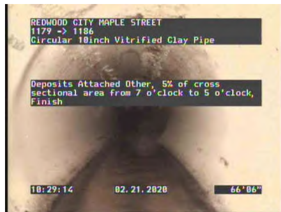
16, 00:07:34, 66.53ft Deposits Attached Other, 5% of cross sectional area from 7 o'clock to 5 o'clock, Finish
