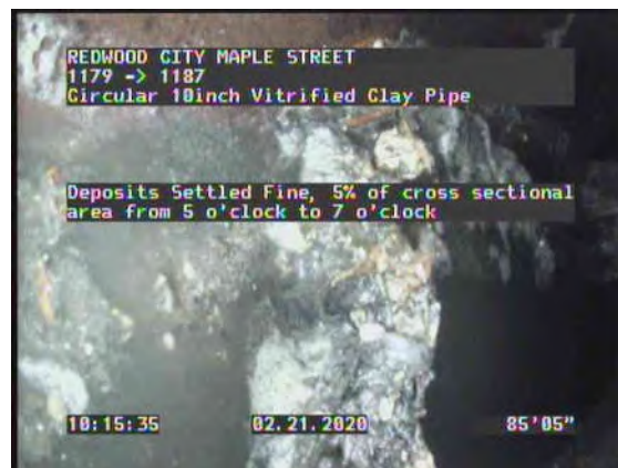
24, 00:08:23, 85.38ft Deposits Settled Fine, 5% of cross sectional area from 5 o'clock to 7 o'clock
