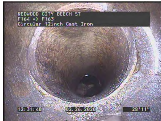
6, 00:02:10, 28.93ft Hole from 10 o'clock to 2 o'clock, within 8 inch
