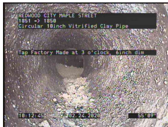
8, 00:04:34, 55.76ft Tap Factory Made at 3 o'clock, 6inch dim
