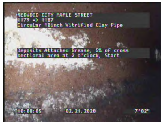
8, 00:02:03, 7.18ft Deposits Attached Grease, 5% of cross sectional area at 2 o'clock, Start
