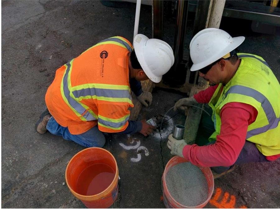
Subject: Typical installation of sacrificial probe for soil gas sampling.
