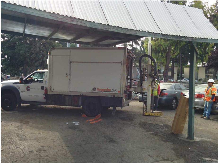
Subject: Set up to drill Boring B4 in the area of the fuel USTs.
