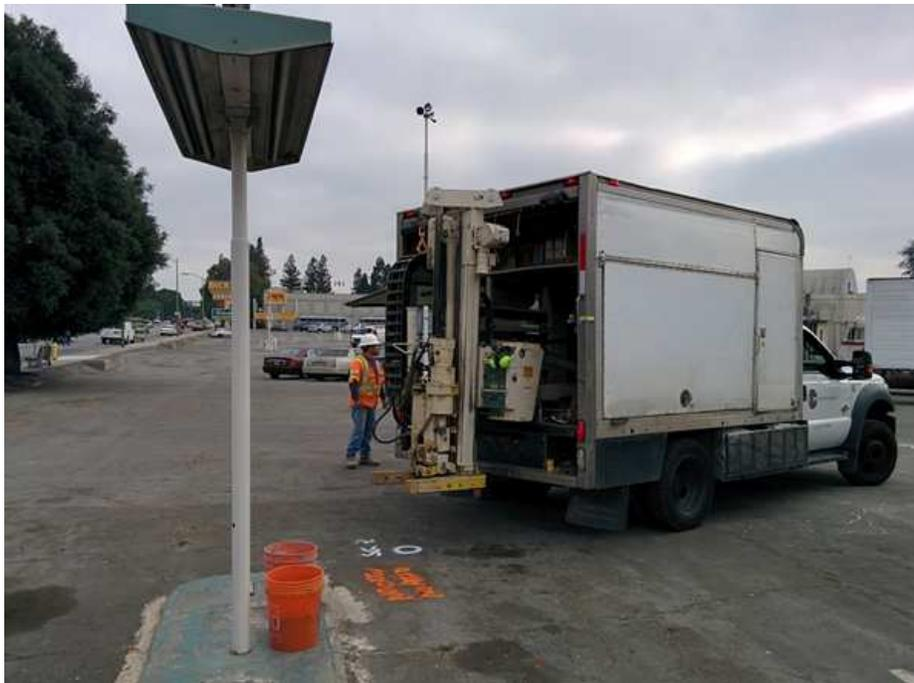
Subject: Preparing to drill boring for soil gas sample SG-2.
