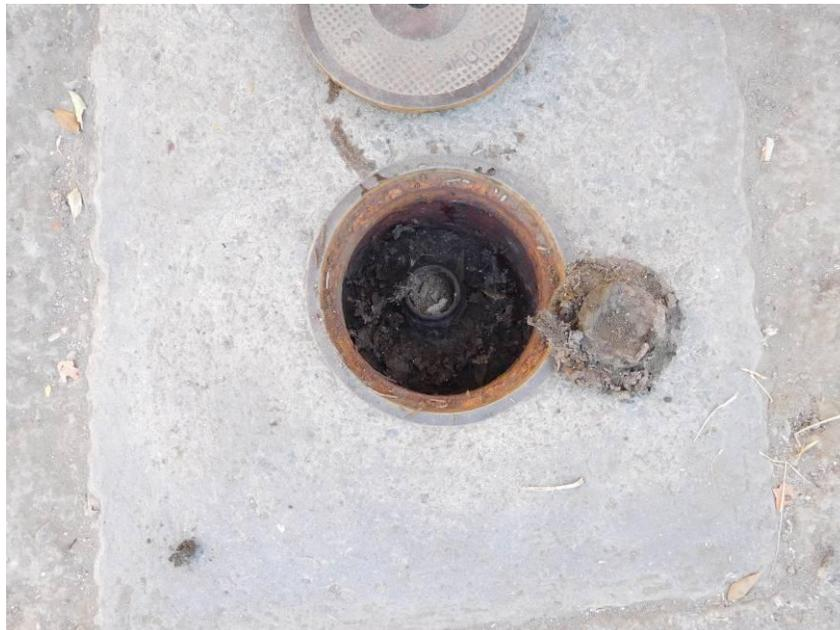
Subject: Subject Property, Fill Box observed on the south side of 1420 South Bascom (the Smog Testing Shop), It appears to be a fill spout for an underground storage tank (UST), filled with sand
