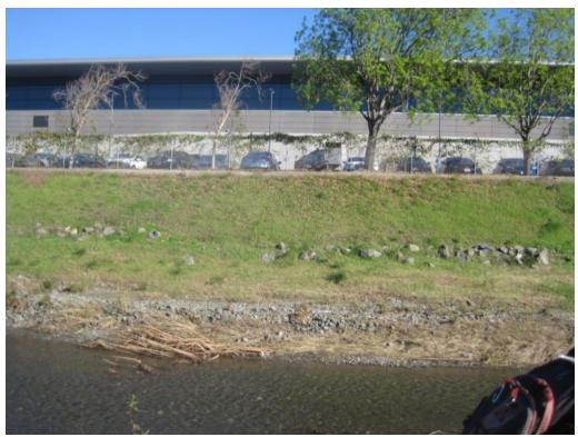
Photo 1. Segment 12, cobble and gravel creek channel supported by light riprap at levee toe (facing west across channel to western access point)
