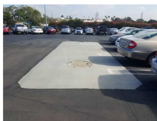
One 10,000-gallon UST is located beneath the existing north surface parking lot on the BCHD campus and is associated with back-up generators located within the attached maintenance building.
