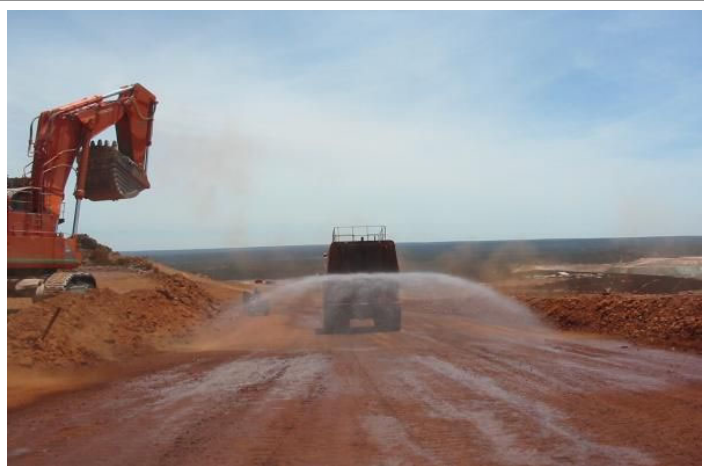
Fugitive dust can be controlled by applying water or other soil stabilizers to exposed soil surfaces daily during construction activities to avoid windblown dust.
