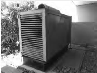
27. Emergency generator with 200-gallon diesel fuel tank adjacent to the 1300 building
