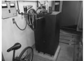
43. 75-gallon diesel fuel day tank for emergency generator in the 1400 building Energy Center
