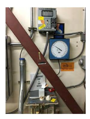
The electronic leak detection and inventory equipment for the underground storage tank behind Building 1400.
