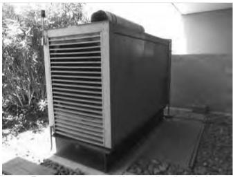
27. Emergency generator with 200-gallon diesel fuel tank adjacent to the 1300 building
