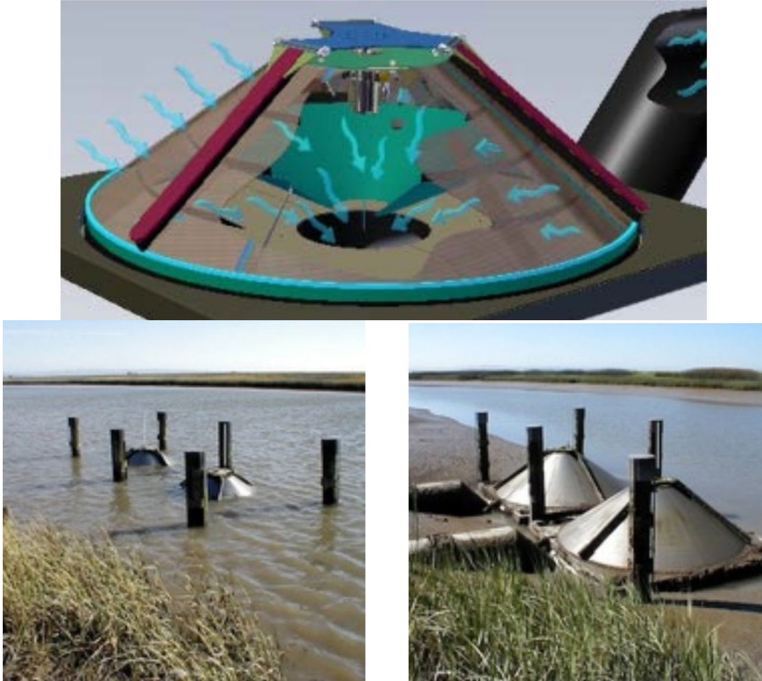
Figure 2-12 Example of Screened Intake
