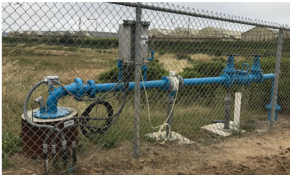
Figure 2-11 Existing Recovery Well
