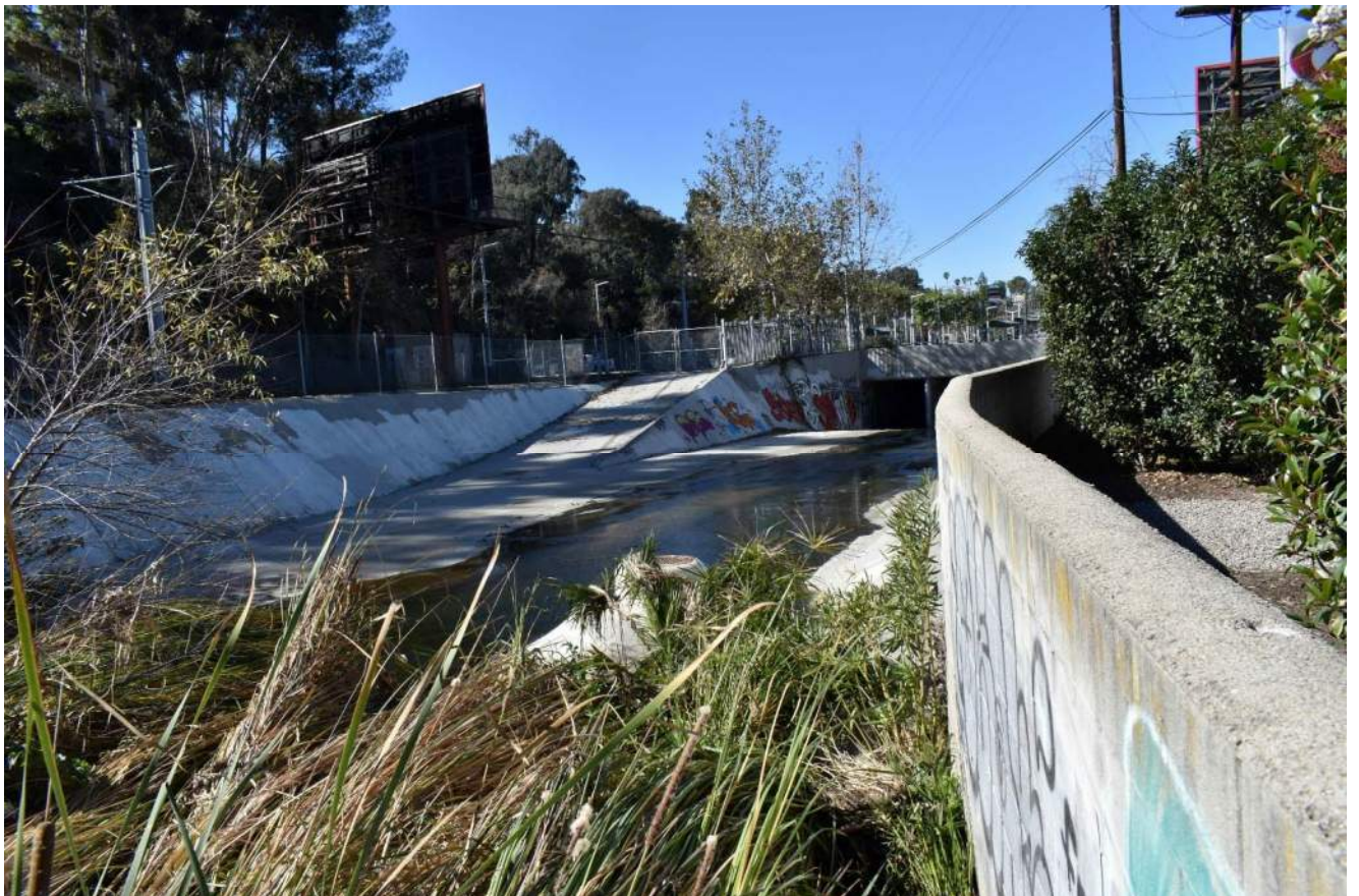
Figure 6. Concrete Channel Lining and Culverts at Lower End of Reach 1
