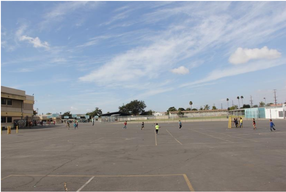
Campus Interior Lacks Shade; Pavement Cracking
