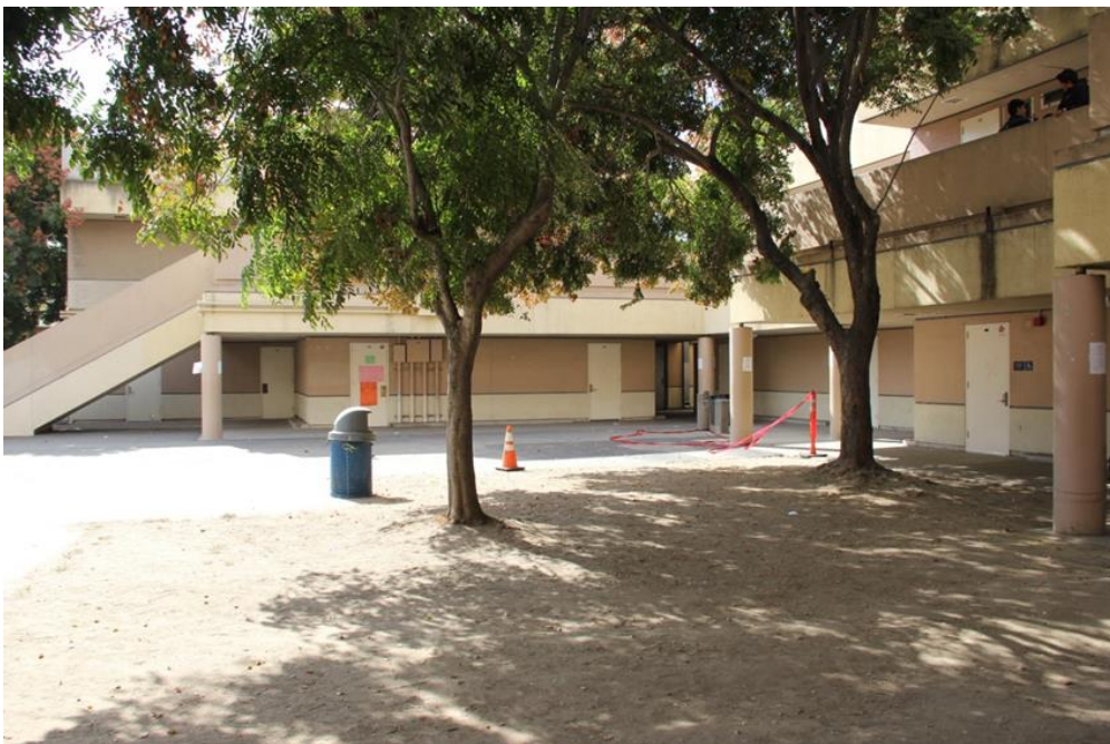
Planting Area Void of Mid-Level Shrub Material
