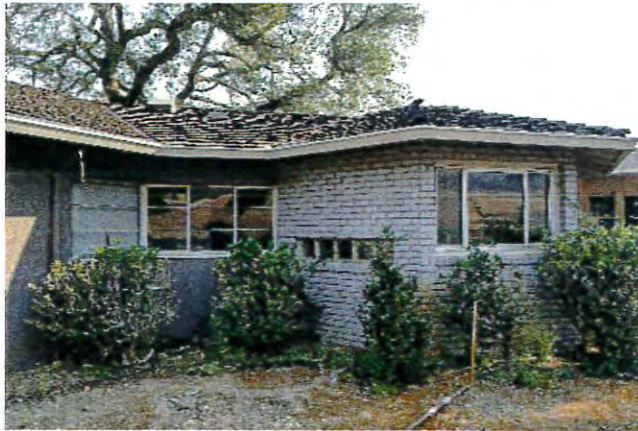
Figure 5: Additional horizontal windows at west façade to north of main entrance. Tripartite window at right is aluminum frame with aluminum casements. Looking north.
