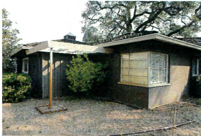
Figure 4: Steel-casement corner window with four divided lites in each section, at west façade. Looking northeast..
