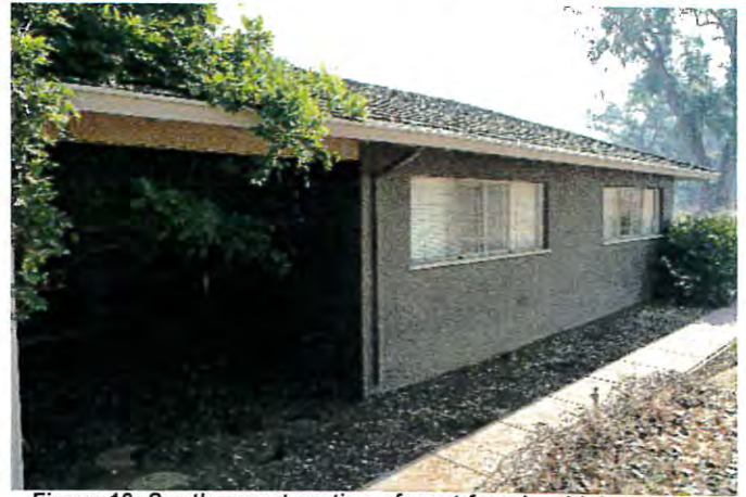
Figure 10: Southernmost portion of west facade which contains two similar aluminum sash sliding windows.
