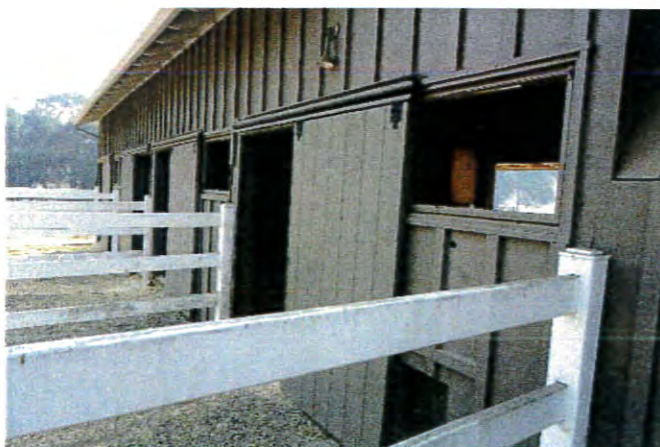
Figure 26: Detail view of horse stalls with sliding wood doors and unglazed windows. Looking southeast.
