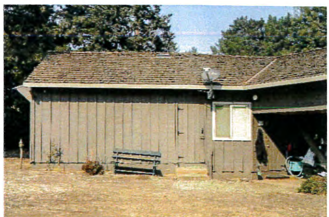
Figure 27: Board and batten siding at south end of barn and stables. Looking west.
