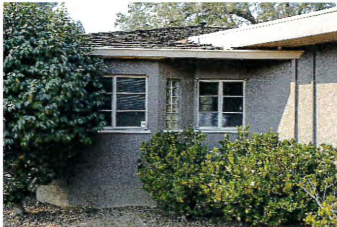
Figure 12: Steel casement windows and column of glass block at east façade. Looking south.
