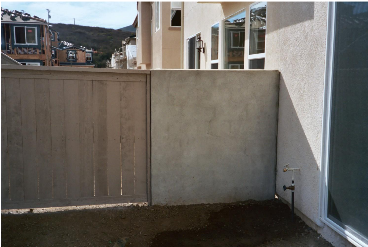
Photo 8: An example of a non-combustible transition between wooden fencing and the structure.
