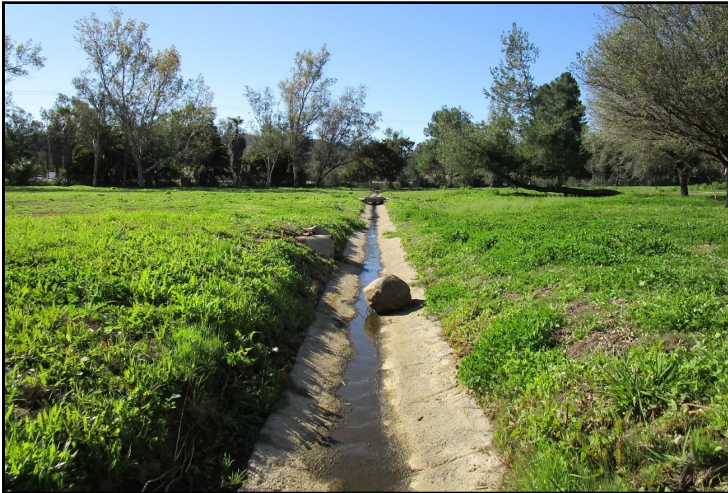
PHOTOGRAPH 5 Concrete-lined Drainage Channel Occurring in the Southwest Portion of the Property
