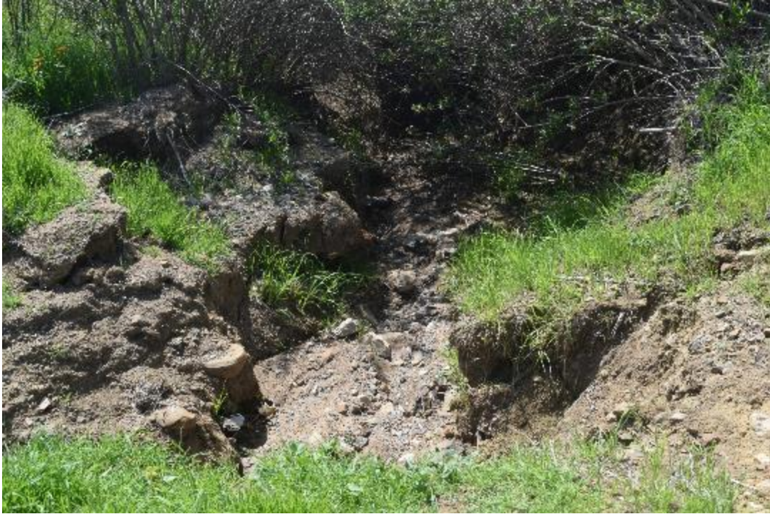
Photo 9. View from the south side of the access road, facing downstream from within Feature 3. This knickpoint is causing additional scouring downstream of the road (refer to Photo 8).
