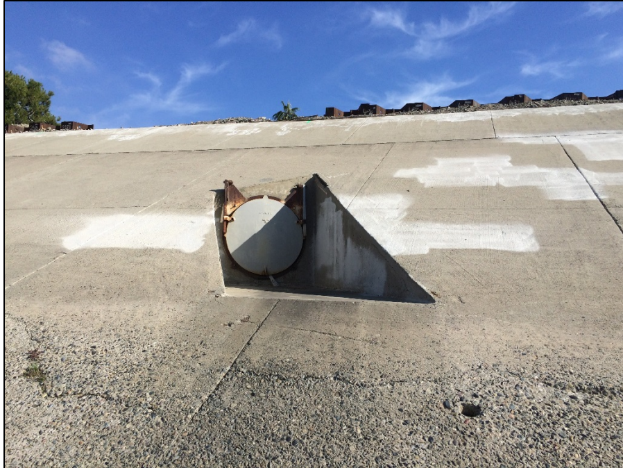
Photograph 3 – 4-foot culvert in northwest project site exit into San Juan Creek
