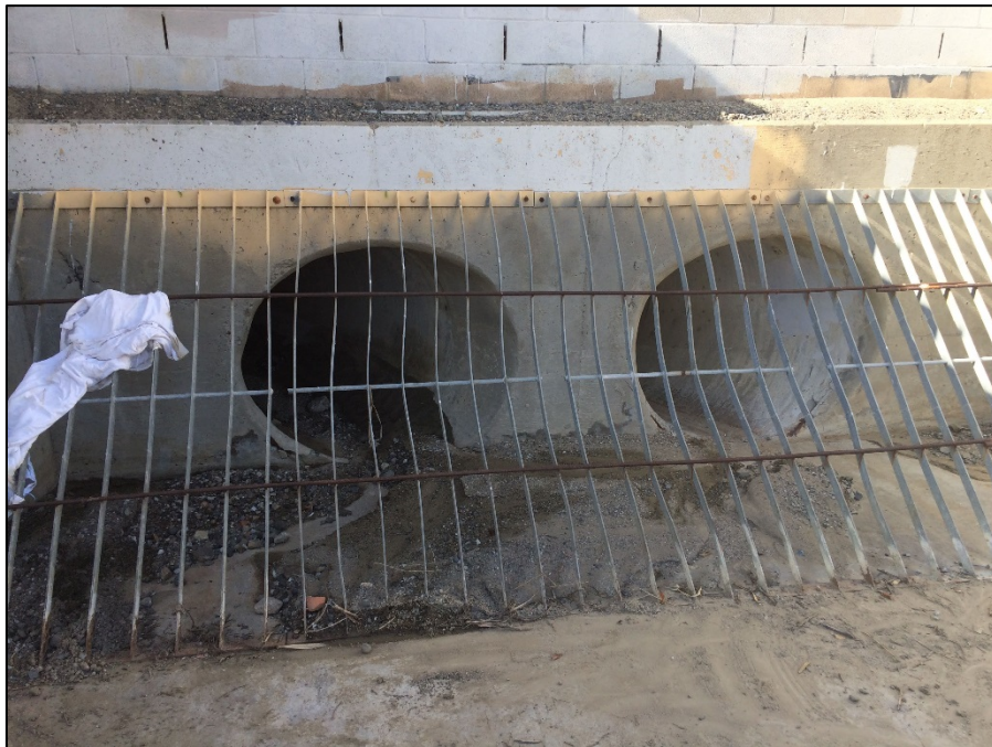
Photograph 4 – Double Culvert in Central-west portion of project site
