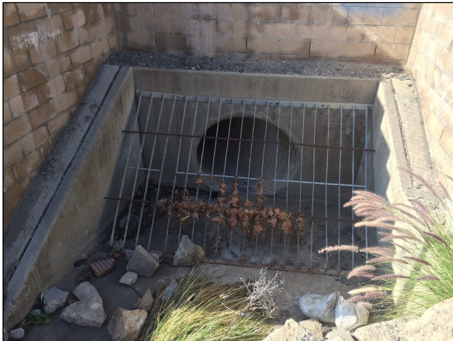
Photograph 2 – 4-foot Culvert exiting site in northwest portion of site
