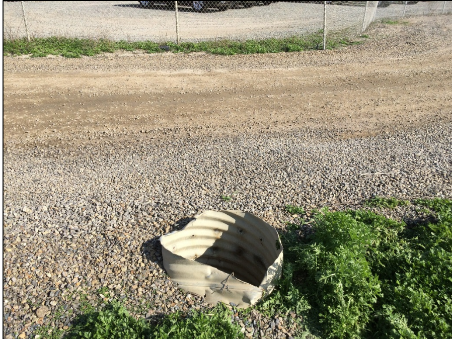
Photograph 13 – One-foot diameter standing pipe within project site
