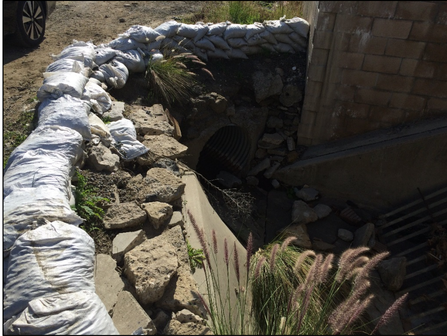
Photograph 1 – Steel Corrugated pipe exiting into 4-foot Culvert in northwest portion of project site
