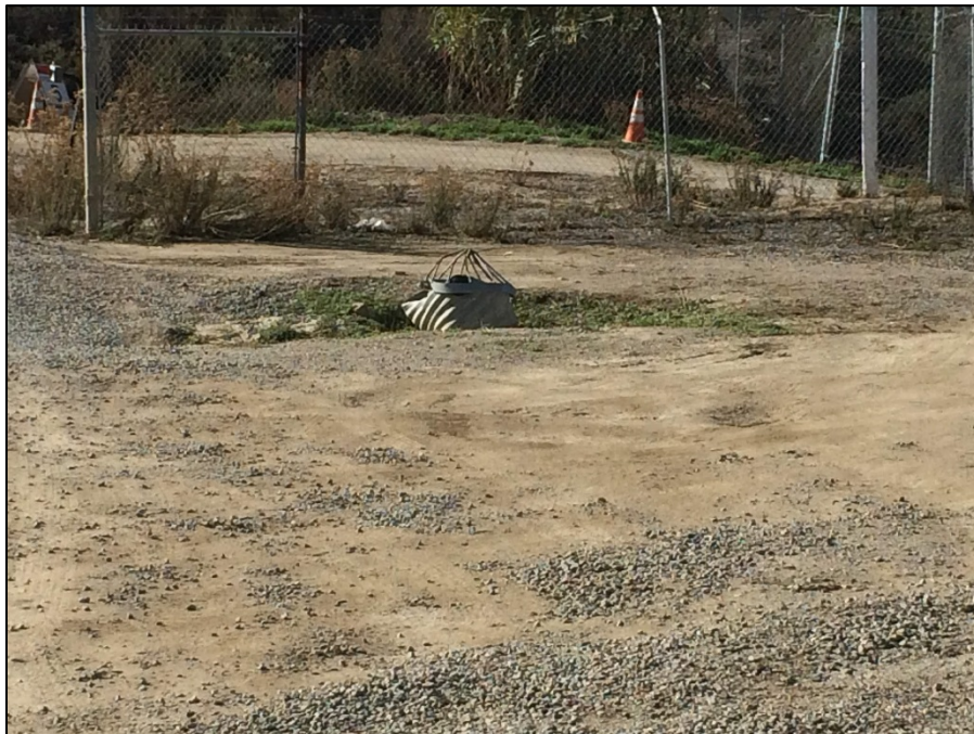
Photograph 14 - One-foot diameter standing pipe within project site
