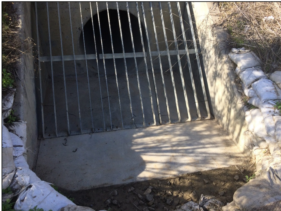
Photograph 6 – 4-foot Culvert in southwest portion of project site
