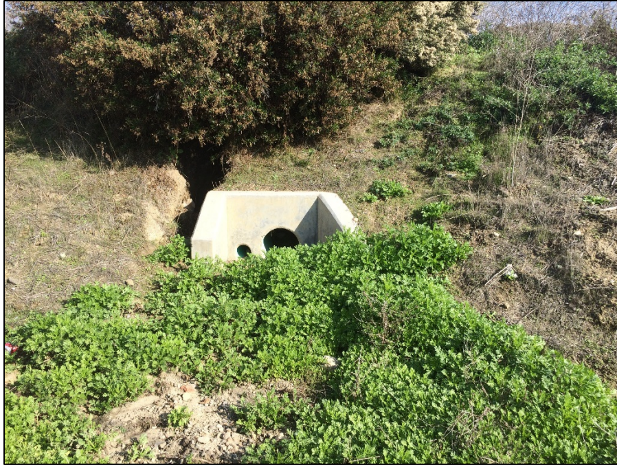
Photograph 11 – Side Culvert to main ditch, draining parking lot
