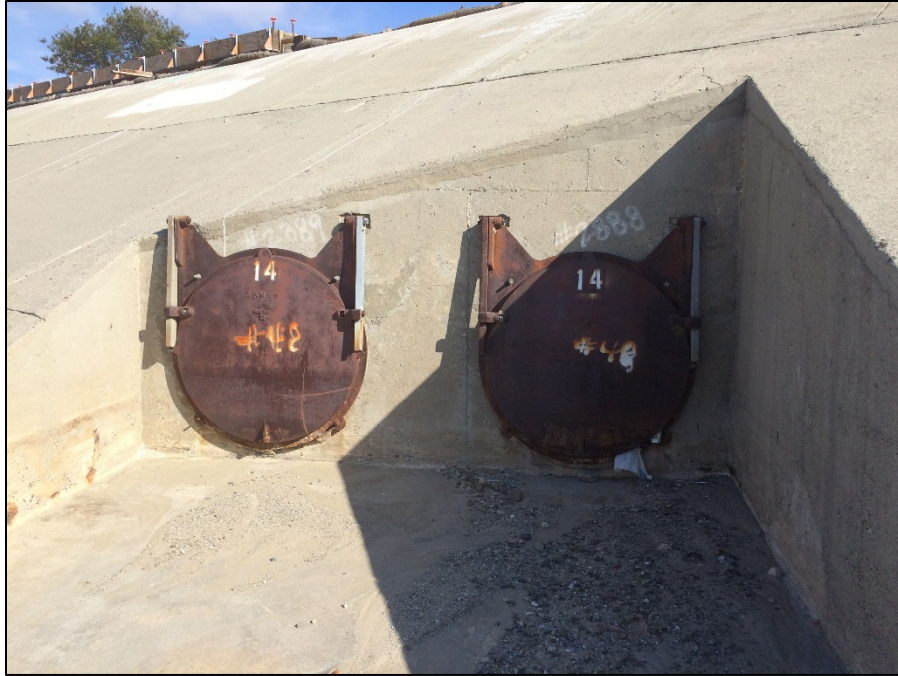
Photograph 5 – Double Culvert exit into San Juan Creek
