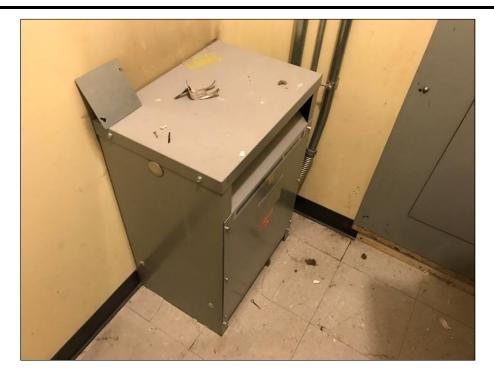
Photograph No. 19 Typical dry transformer located throughout the interior of site buildings.
