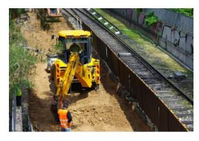
A construction barrier is built at the edge of the site to protect tracks from adjacent work.
