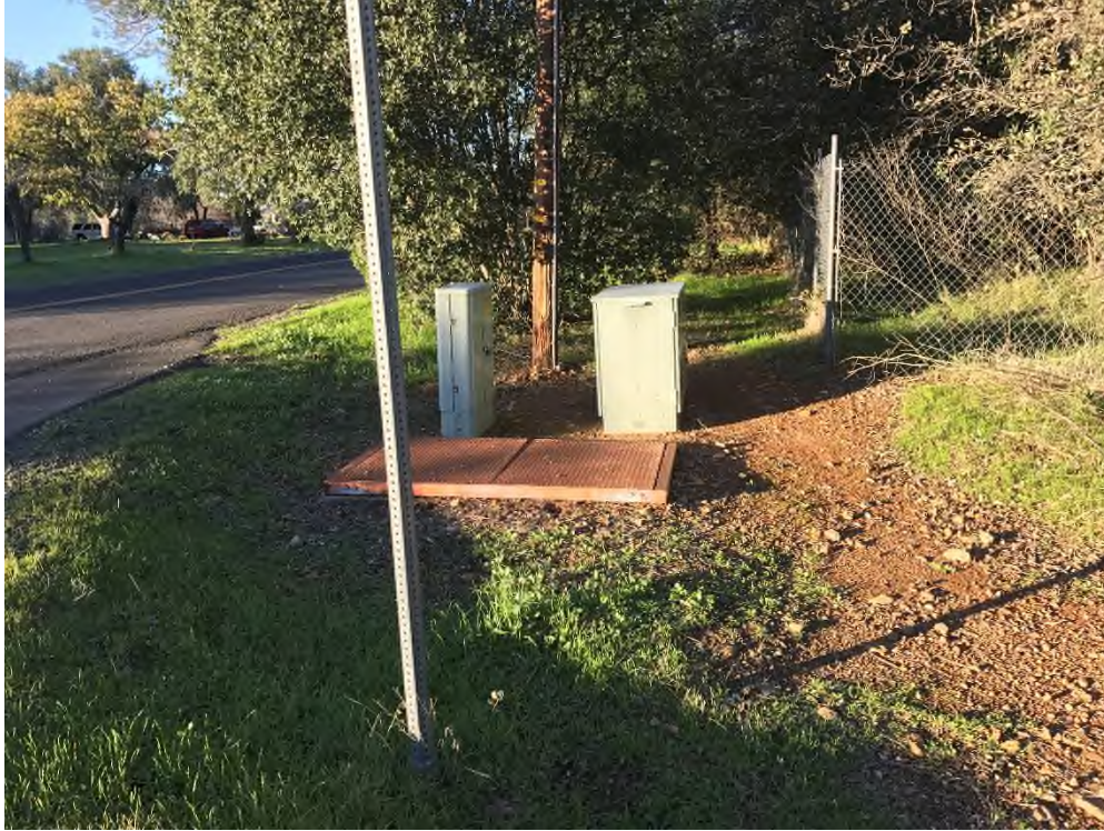
Photo 1. One of the six existing DLC sites for the Proposed Project that is proposed for renovation. This DLC site is located alongside (in the shoulder of) an existing public road. A brown metal trapdoor, in the center of the photograph, covers the existing underground vault at this DLC site. The putty-colored aboveground metal equipment cabinet to the right and the smaller, putty-colored cross-connection box to the left are located next to the buried vault at this site, instead of on top of the vault. A small graveled area is surrounds the aboveground components of this DLC site. Roadway signposts (foreground) and a telephone pole (background) share this area, along with fencing for an adjacent property.
