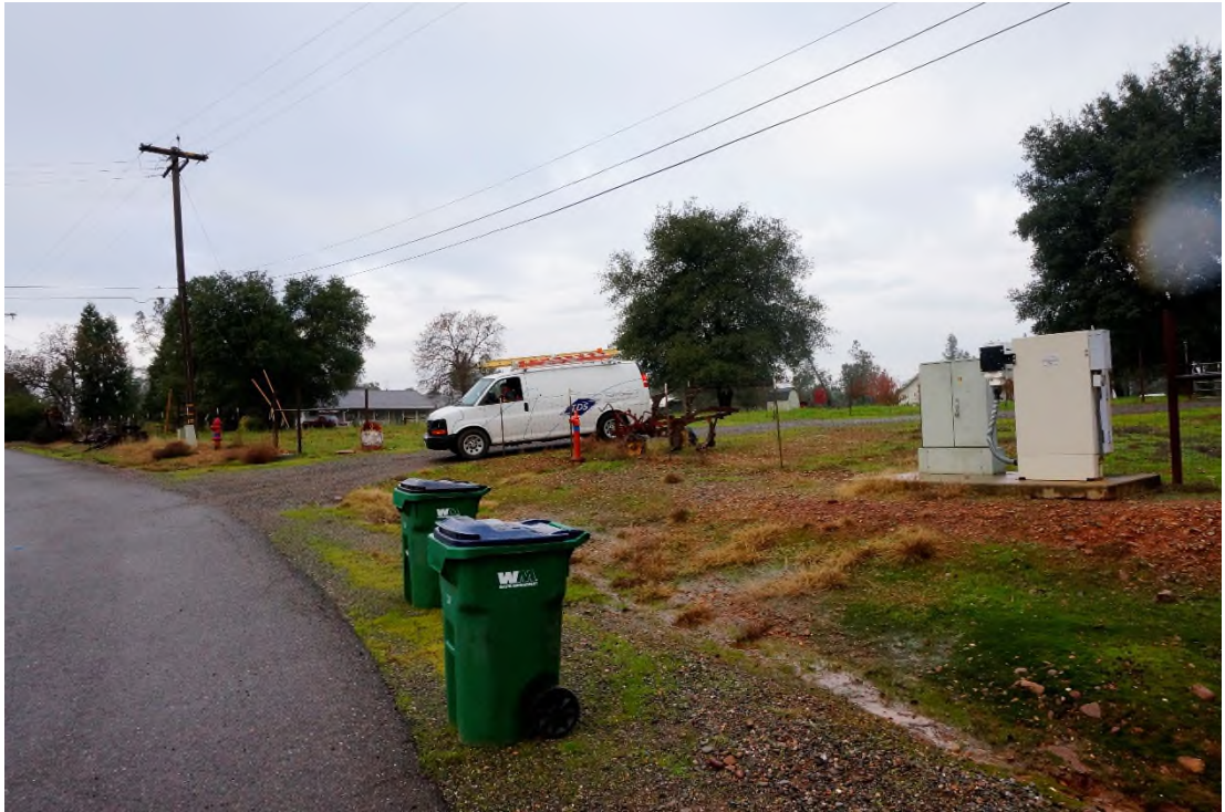
Photo 2. Another of the six existing DLC sites for the Proposed Project that is proposed for renovation. This DLC site is also located alongside (in the shoulder of) an existing public road. The putty-colored aboveground metal equipment cabinet on the right behind the vault and the smaller, putty-colored cross-connection box on the left are located on top of the buried concrete vault at this DLC site. A small graveled area is surrounds the aboveground components of this DLC site. A telephone pole (background) and visible overhead wires share this area, along with fencing for an adjacent property.
