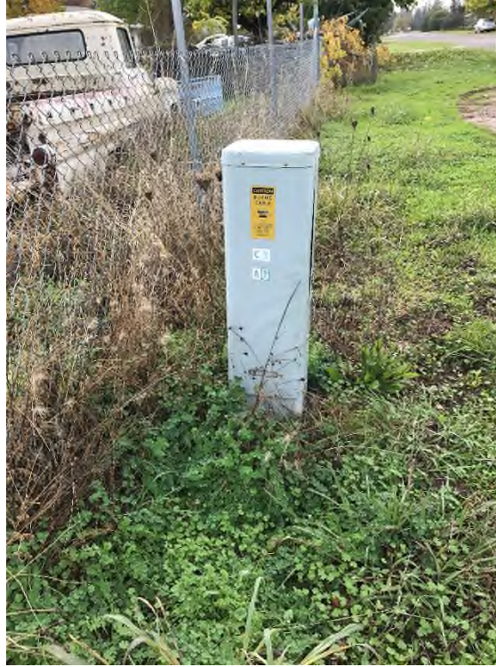
Photo 5. An example of an existing cross-connection box that would be installed at each of the seven new DLC sites and at any of the six existing DLC where renovation activities would include replacement of the existing aboveground cross-connection box.
