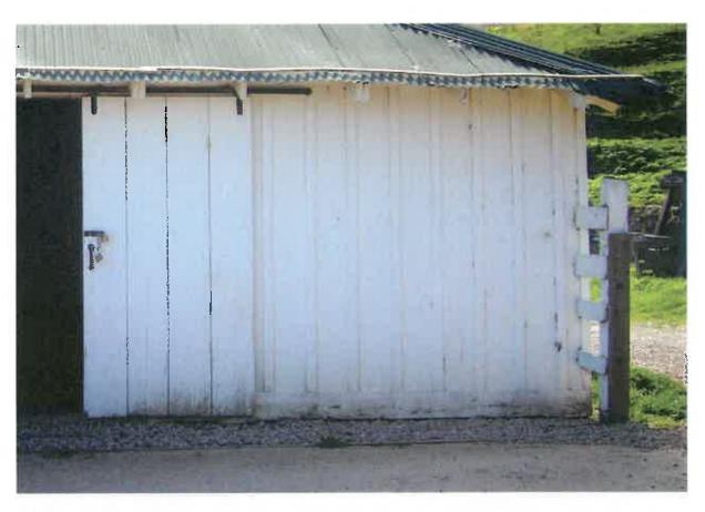
Figure 46. Soiling at the base of the exterior siding.
