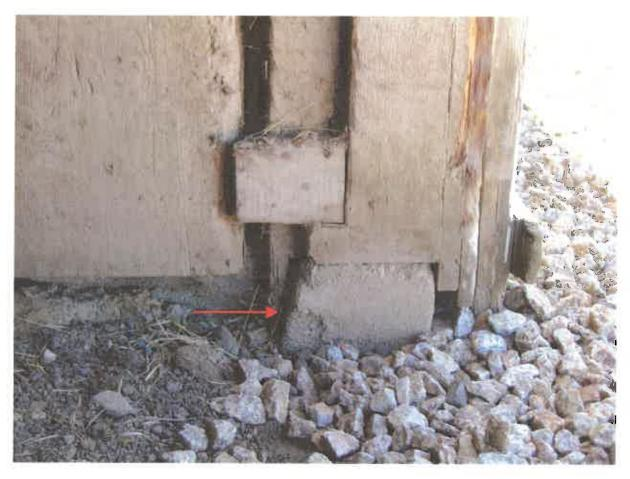
Figure 45. Subgrade perimeter foundation at the west elevation.
