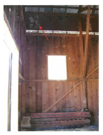
Figure 64. Water stains on the wood boards at the northeast corner of the center aisle. And old rail track stored on the fragile floorboards in the center aisle.
