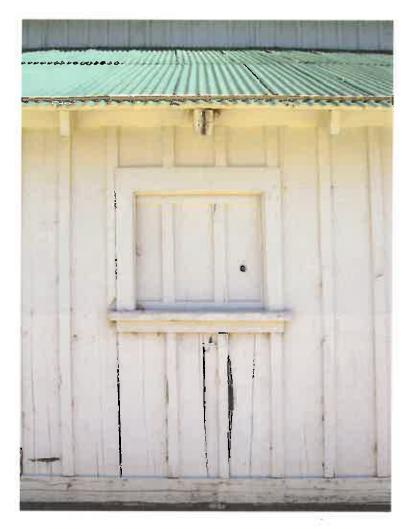
Figure 23. Typical sliding window at the west elevation.
