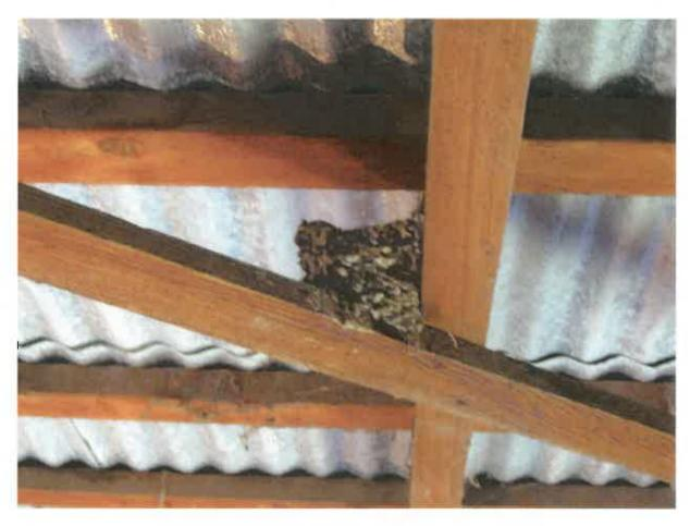
Figure 62. Bird nest found nestled within roof framing system at the center aisle.
