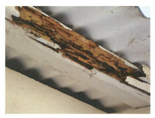
Figure 60. Detail view of deterioration at sleepers.
