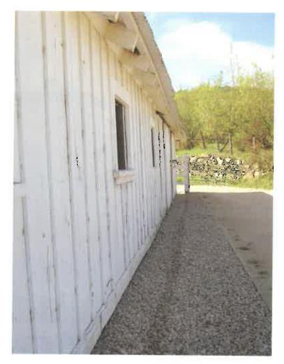
Figure 9. French Drain at the west elevation.
