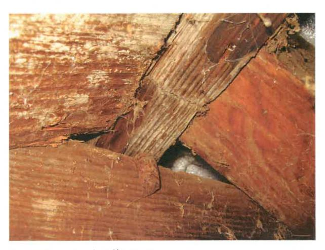
Figure 56. Deterioration at the roof framing system.
