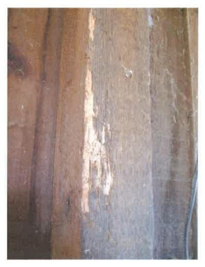
Figure 53. Typical surface deterioration from insect infestation at the timber posts.
