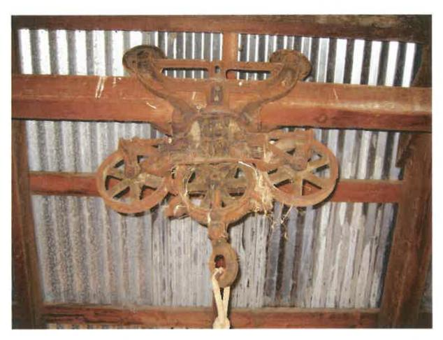
Figure 66. Hoist at the center aisle used to transfer hay in and out of the Fish Lower Barn. The hoist rides along the square beam hung from the ridge beam above.
