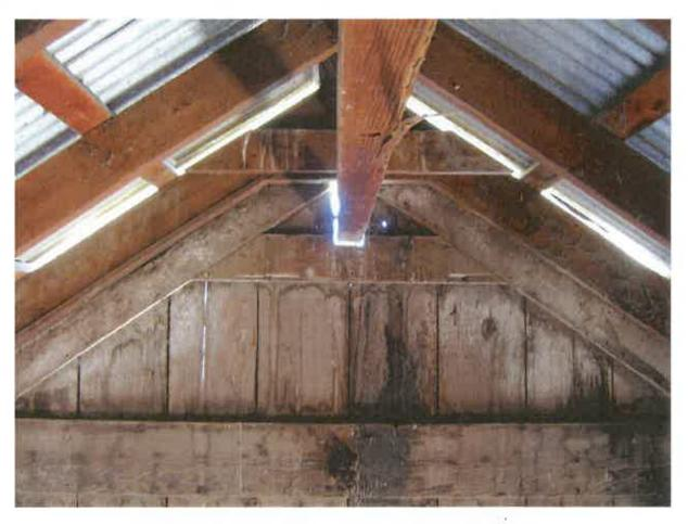
Figure 52. Watermarks found throughout the interior face of the wood siding.
