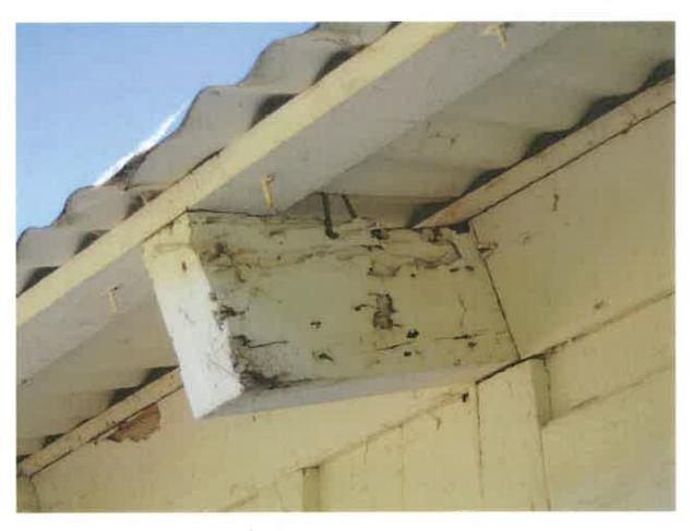
Figure 58. Typical deterioration of roof rafter ends.
