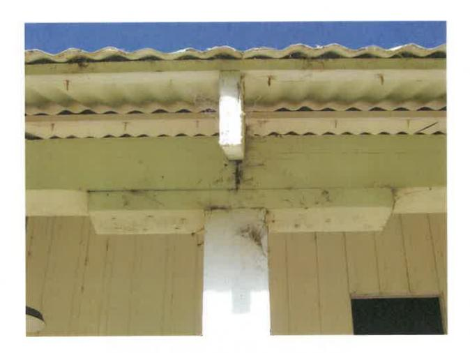
Figure 34. Structural framing system of the east aisle.
