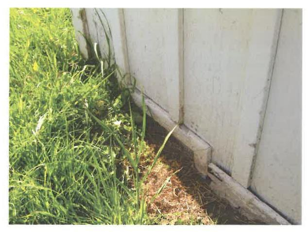
Figure 47. Soiling at the base of the wood siding.
