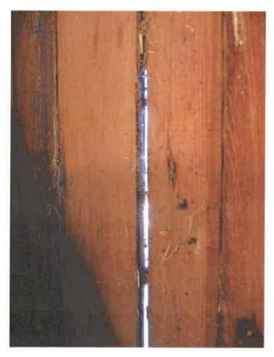
Figure 51. Typical gap between exterior siding.
