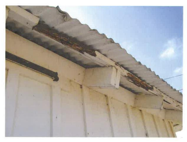
Figure 59. Deterioration of sleepers at roof framing system.
