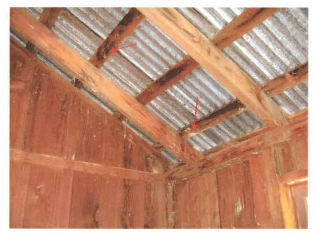
Figure 65. Deterioration of the roof framing system at the rear storage areas.
