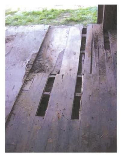
Figure 63. Deteriorated floorboards at the center aisle.
