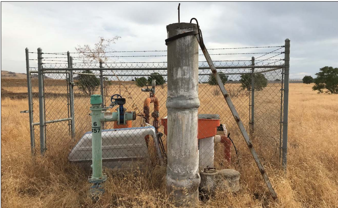
Figure 4-12 Concrete agricultural standpipe and short riser beside modern agriculture pump and fenced enclosure; view to the south.
