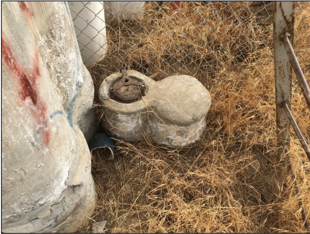
Feature 4 Agricultural riser beside standpipe. (Frame 56).
