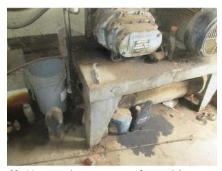
23. Motors and compressors at former dairy, minor oil staining.
