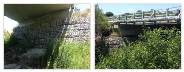
Photo 7 - Gabion Baskets (east bay under bridge) Photo 8 - West Bay of Bridge (upstream view)
