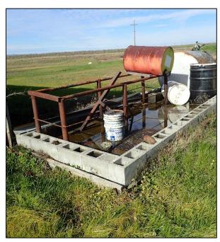
Photo 14. Waste oil collection area with secondary containment (Figure 2a).
