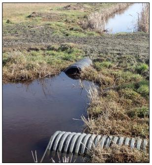
Photo 3. Irrigation culverts with 12-inch diameter corrugated piping. Located parallel to a levee near Malcolm Lane (Figure 2b).
