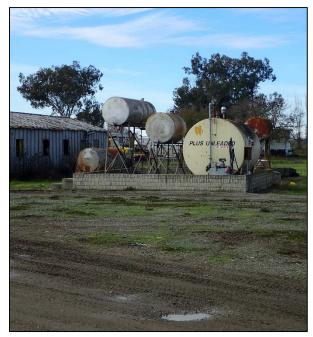
Photo 20. 5,000 gallon unleaded gasoline AST on concrete foundation (secondary containment, Figure 2a).
