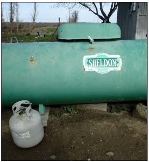
Photo 31. 250 gallon LPG AST tank associated with mobile residence (Figure 2a).
