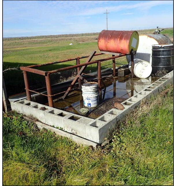
Photo 14. Waste oil collection area with secondary containment (Figure 2a).
