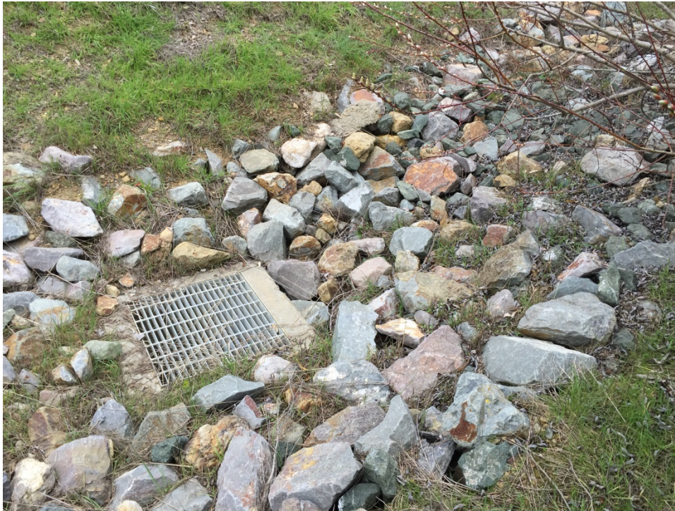
Photograph 5: The culvert at the western end of the swale.
