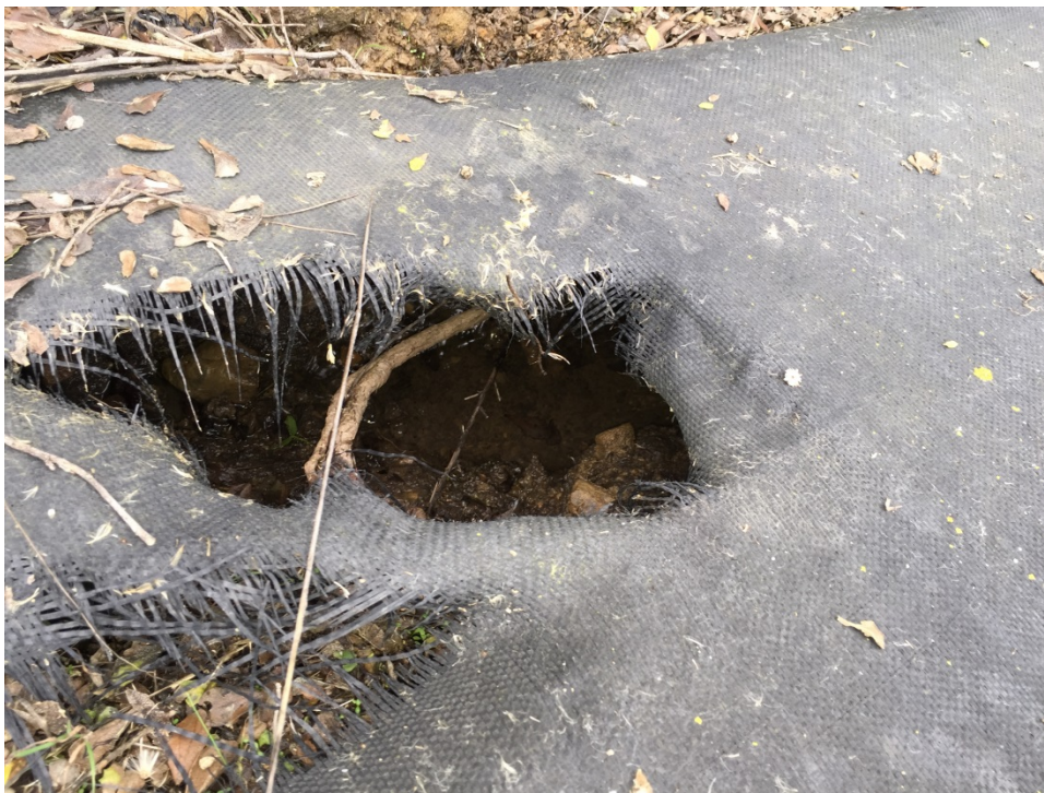
Photograph 4: Water flowing under disintegrating plastic sheeting in the swale at the north end of the property
