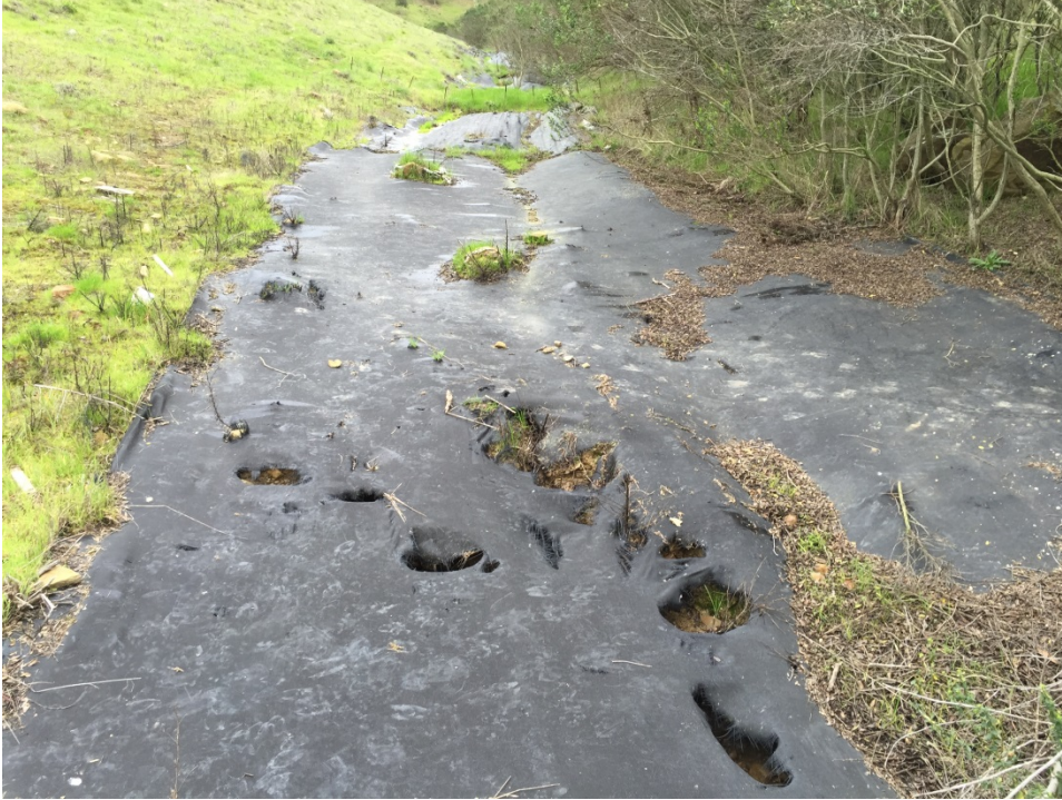
Photograph 7: Raccoon and deer prints on the degraded plastic sheeting in the swale on the north side of the property
