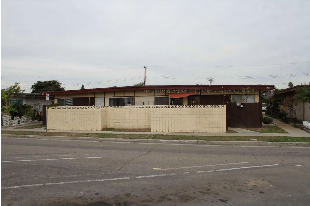
Figure 16: View looking north across W. Pacific Avenue at the apartment at 8921 W. Pacific Avenue, which retains most of its original design elements, including the batten stucco exterior wall cladding and window fenestration, and concrete block walls.
