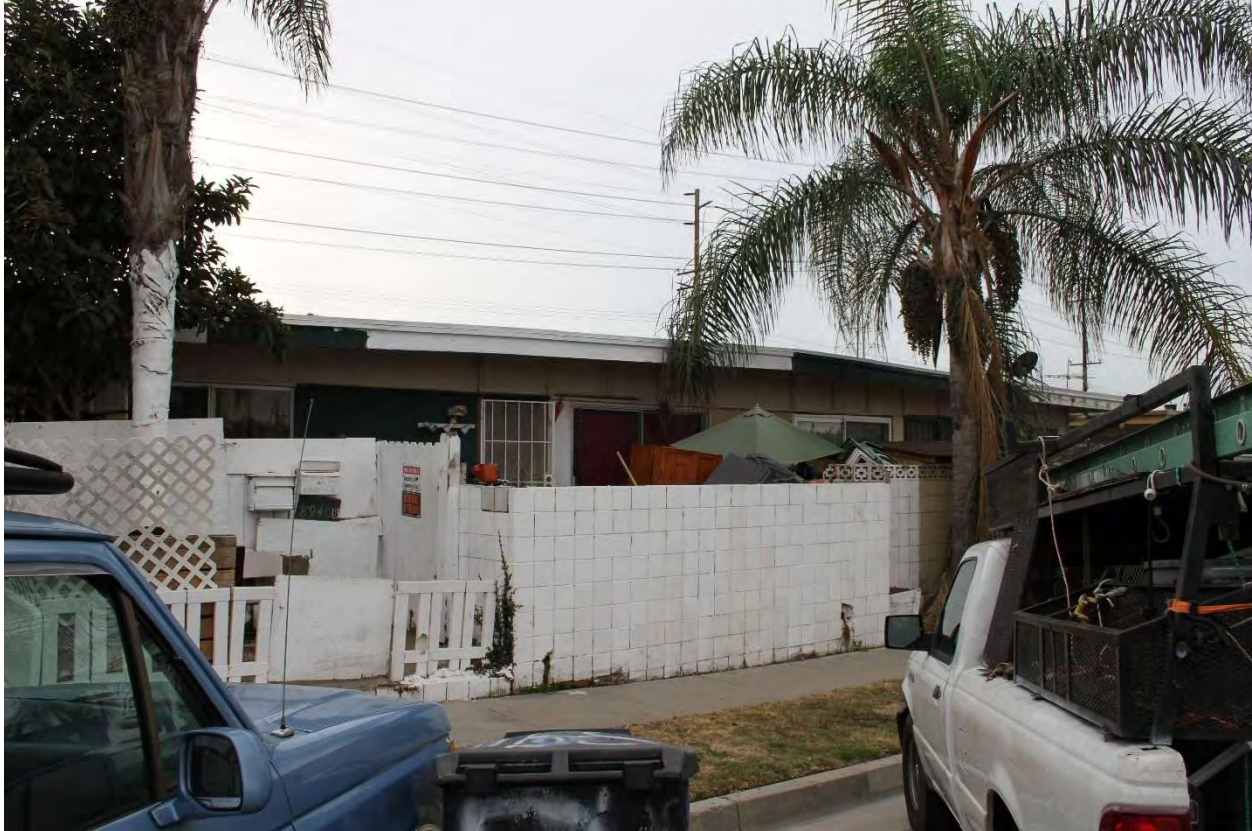
Figure 15: View looking southwest at the four-plex at 8940 W. Pacific Avenue. Note the alteration to the original concrete block walls fronting the apartment, along with numerous window alterations and the addition of a security screen door.
