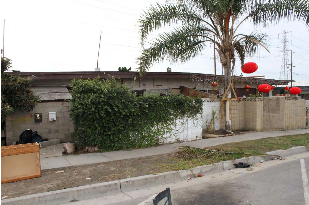
Figure 14: View looking southwest at the four-plex at 8970 W. Pacific Avenue. Note the contemporary concrete block wall on the left of the photograph and the original concrete block wall on the right with decorative trim blocks. This unit appears to have its original batten exterior wall siding and many of its original aluminum slider windows.
