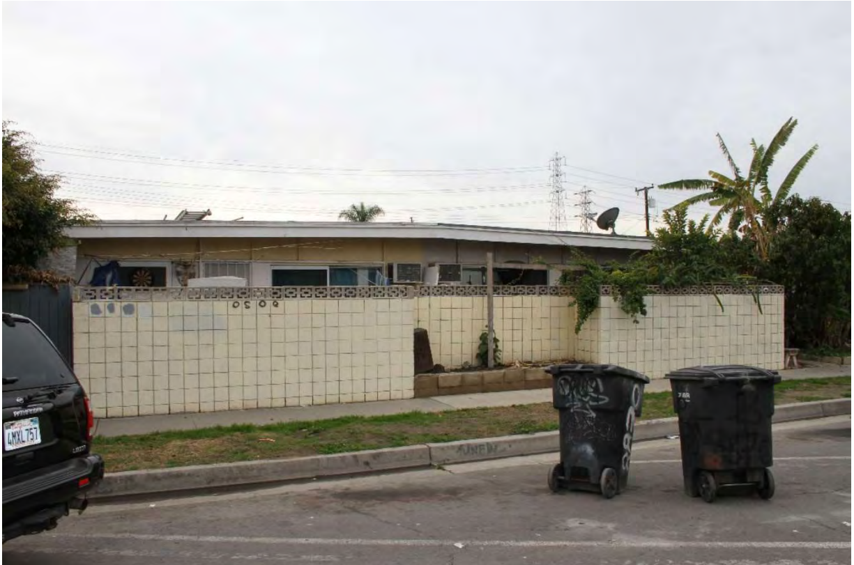
Figure 26: Tina-Pacific four-plex nearly identical to the Huntington Beach model in Figure 25, with a similar roof design and exterior wall battens. Note that the decorative openwork or geometric concrete blocks atop the privacy wall are missing from the Huntington Beach model.
