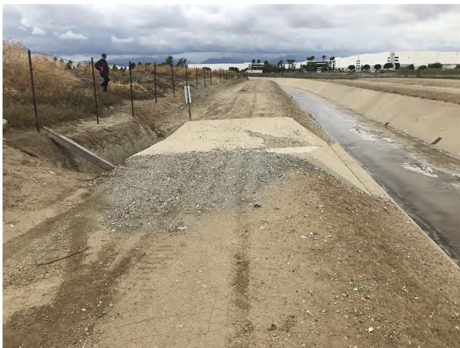
Photograph 5: Photograph depicting Cypress Channel. Note the concrete sides and bottom.
