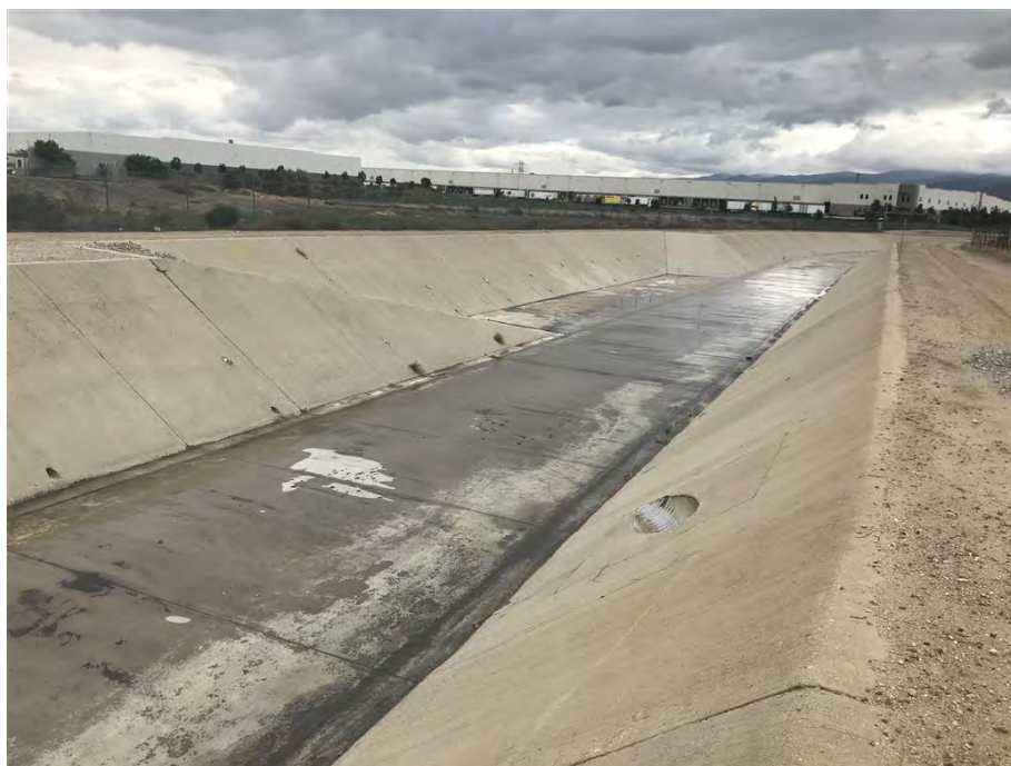
Photograph 6: Photograph depicting Cypress Channel. Note the concrete sides and bottom.
