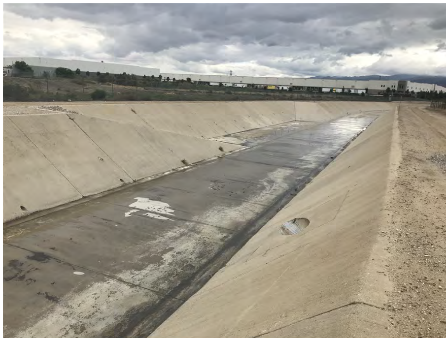
Photograph 22: Photograph depicting Cypress Channel. Note the concrete sides and bottom.
