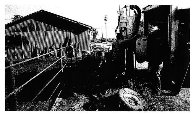
BORING H4 23.5' SOUTH OF H3, 81" EAST OF STEEL FENCE, IN DIRT EAST OF CONCRETE APRON. TOTAL DEPTH 39'. GROUNDWATER MOIST AT 30'; WET AT 36.5'; TOTAL DEPTH = 39'. LOOKING AT NORTH TOWARD PINE AVE.
