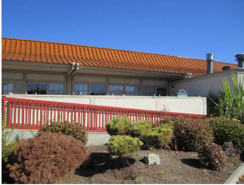
Figure 5 West elevation. Photo taken Nov 12, 2015
