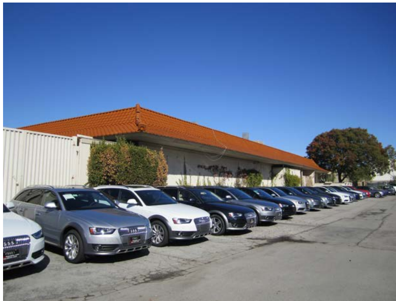
Figure 6 South (Rear) elevation. Photo Taken Nov 12, 2015
