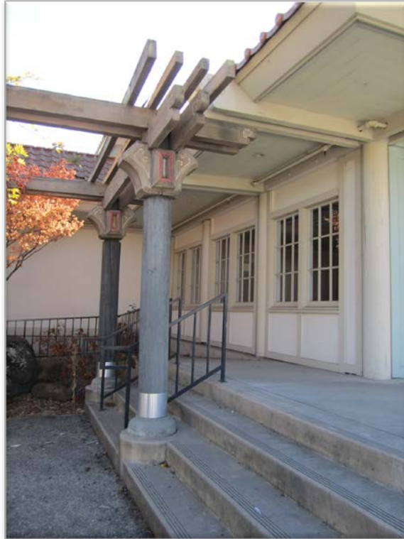
Figure 3 Close Up of Architecture at Northeast corner. Photo Taken Nov 12, 2015
