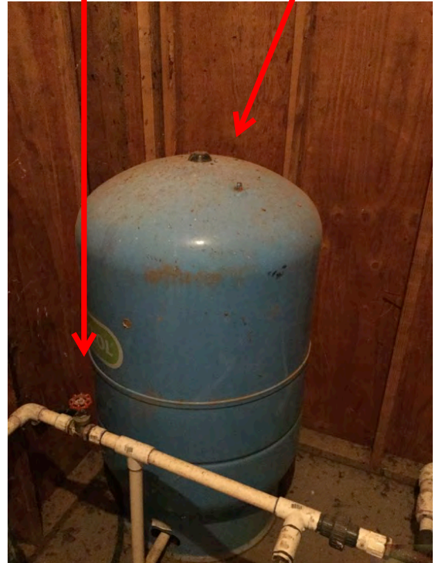
Main Shut-off 86 Gallon Pressure Tank
