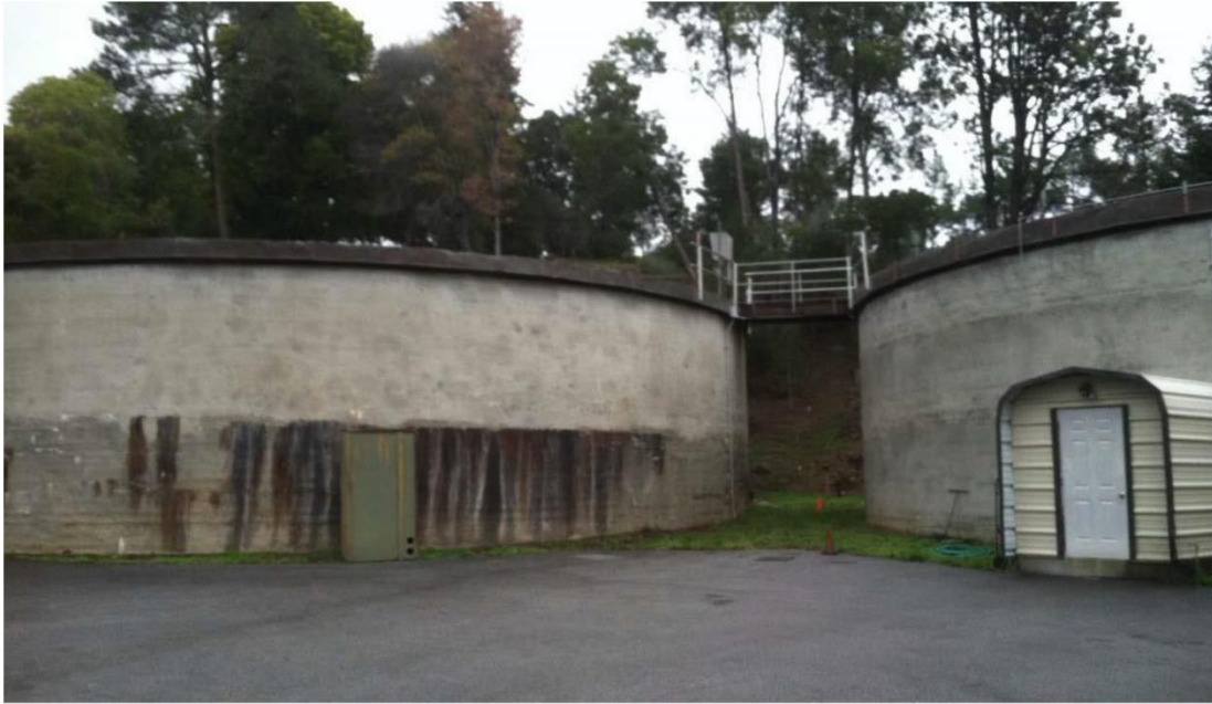
Existing Sludge Storage Tank with Horizontal Staining Line from Leaks
