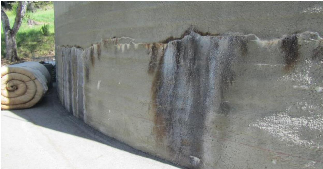
Close Up Photo of the Sludge Storage Tank with Horizontal Staining Line
