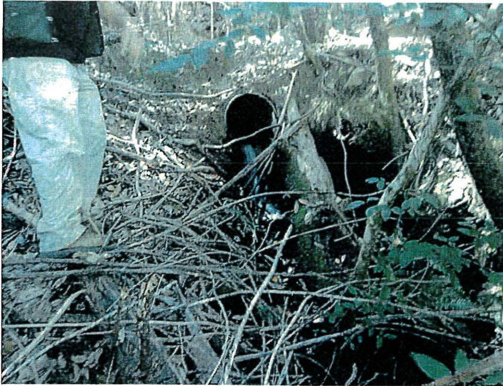
Photo 29. LSAA Project 2, looking upstream at outlet. Note undercutting. July 26, 2017
