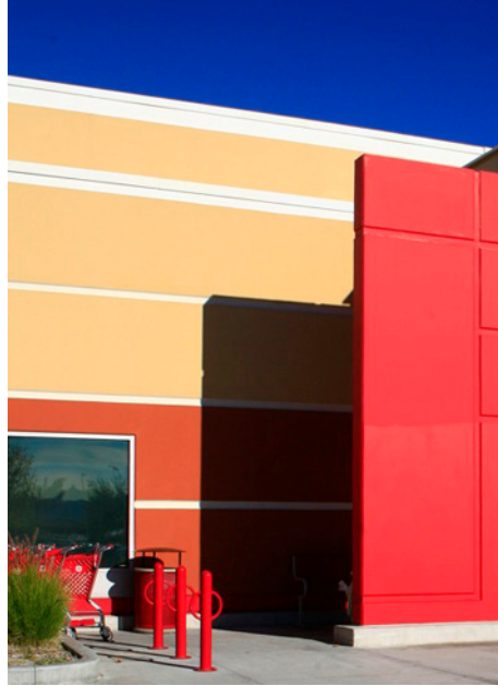
Painted tilt up concrete panels
