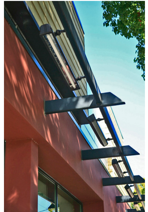
Metal Shade Elements Supporting Lighting
