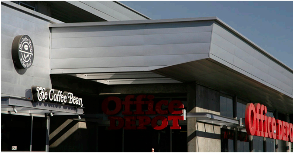
Interlocking horizontal metal panels
