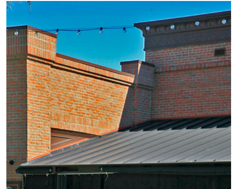
Brick walls with standing seam metal roof
