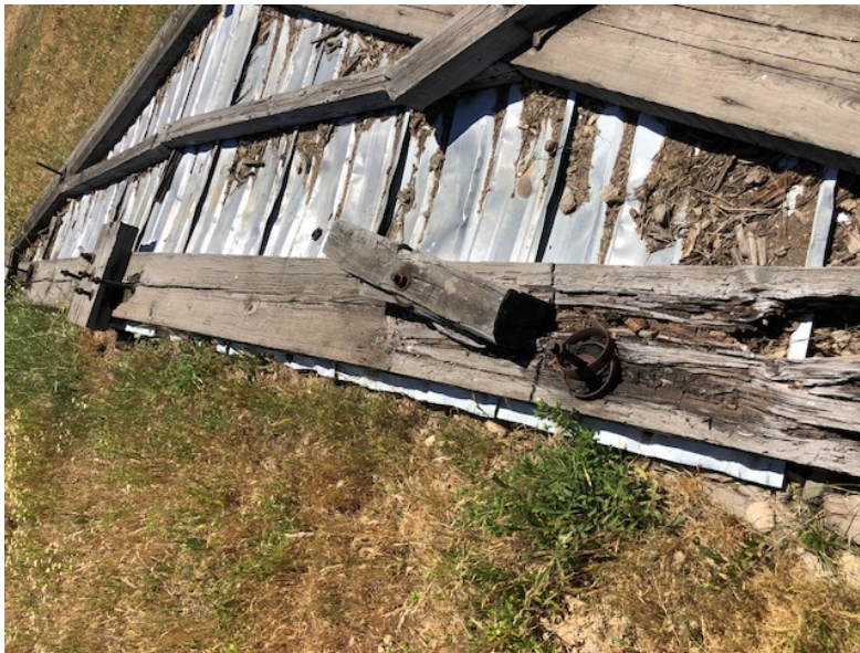
Intact truss construction detail. Note shear ring for construction.
