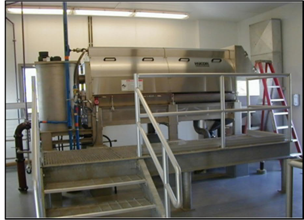
Figure 5-12 – Rotary Drum Thickener Illustration
