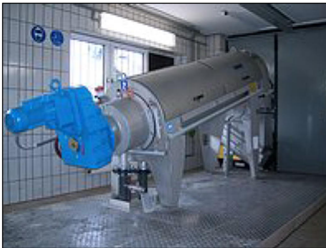
Figure 5-18 – Screw Press Illustration
