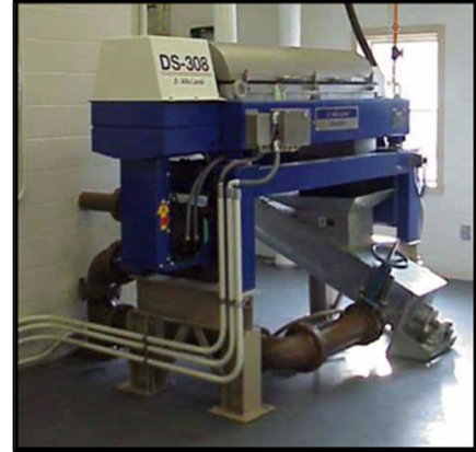
Figure 5-16 – Centrifuge Illustration
