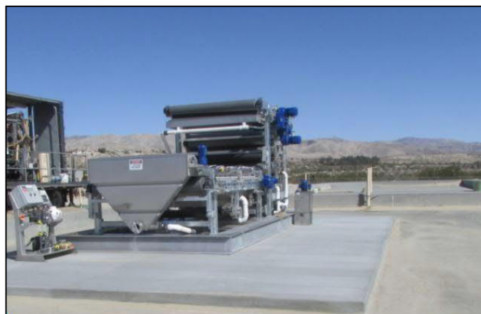
Figure 5-15 – 3-Belt BFP Illustration
