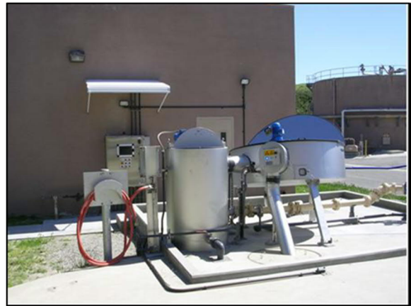
Figure 5-13 – Disc Thickener Illustration
