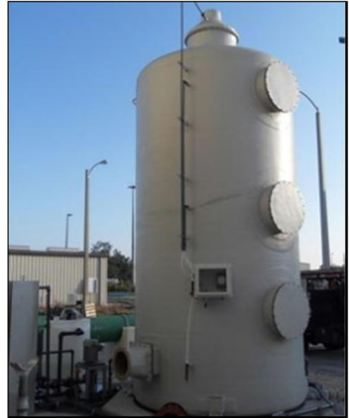
Figure 5-21 – Biotrickling Filter Illustration
