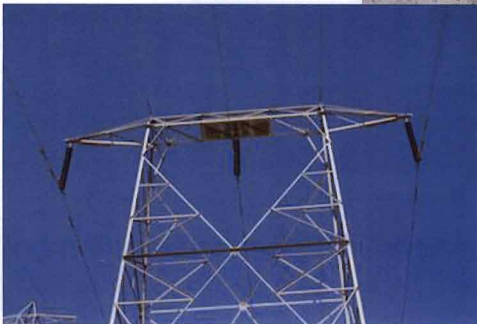
Detail of extant porcelain insulators at Mile 39 Tower 3. Photo Credit: Steven Treffers, SWCA Environmental, Inc.
