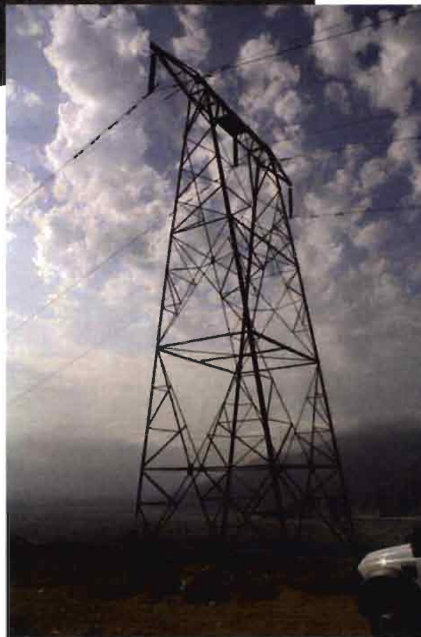
View southeast of Mile 64 Tower 4, an original Type S Suspension Tower, on the western side of Whitewater Canyon. Photo Credit: Steven Treffers, SWCA Environmental, Inc.
