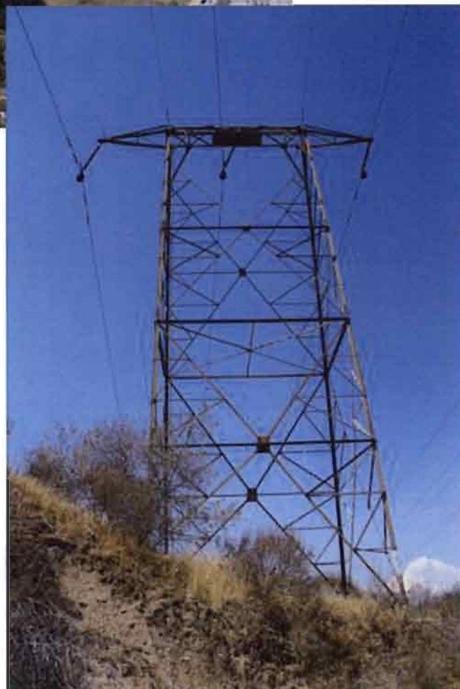
View west of Mile 99 Tower 2. This is the last original tower type, believed to be an L Type, at the western end of Devers-San Bernardino 220kV Transmission Line where the historic-era Chino-Hayfield alignment continues on as the replaced non-historic portion of the Devers-Vista No. 1 220kV Transmission Line. Photo Credit: Steven Treffers, SWCA Environmental, Inc.
