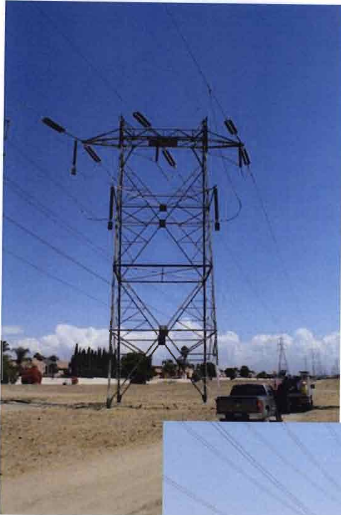
View northeasterly of a Transposition Tower at Mile 9 Tower 4. Photo Credit: Steven Treffers, SWCA Environmental, Inc.
