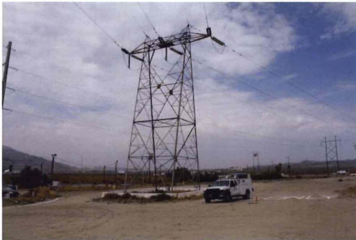
View southwest of Mile 74 Tower 1, an original Type D Dead End Tower. Photo Credit: Steven Treffers, SWCA Environmental, Inc.
