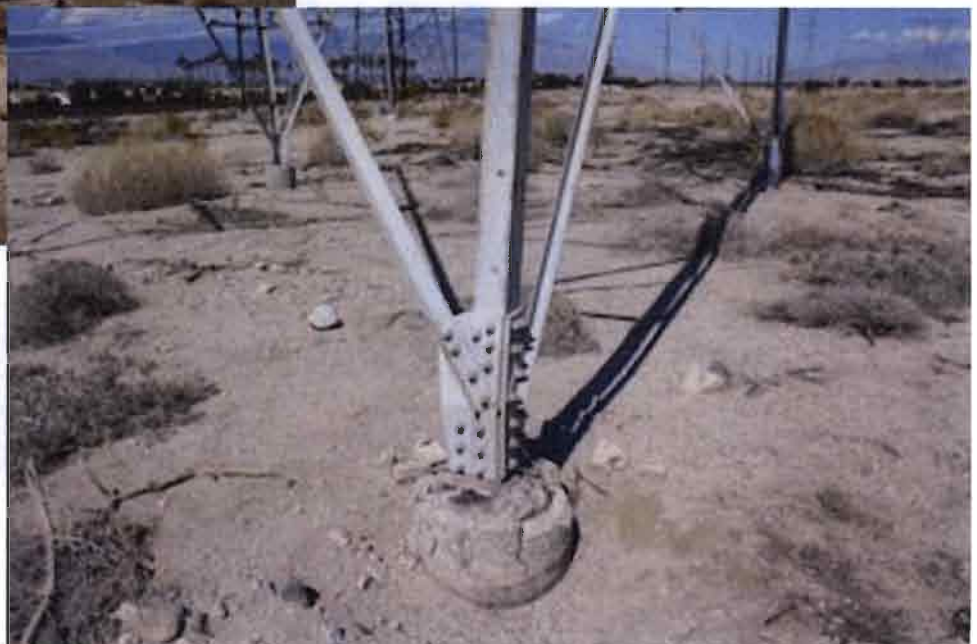
Detail of the northeast tower concrete footing at Mile 40 Tower 2. Photo Credit: Steven Treffers, SWCA Environmental, Inc.
