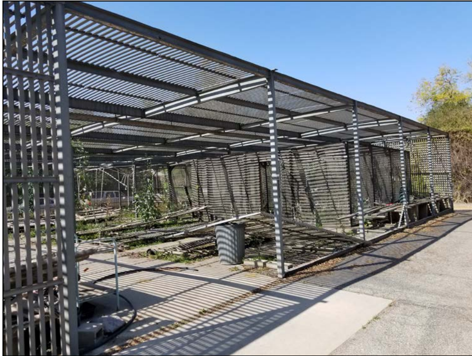
Detached siding on north-facing façade of lath house and interior screen house, facing southwest.
