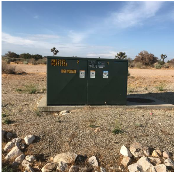
Photo #5 Pad-mounted transformer in north-central portion of site.
