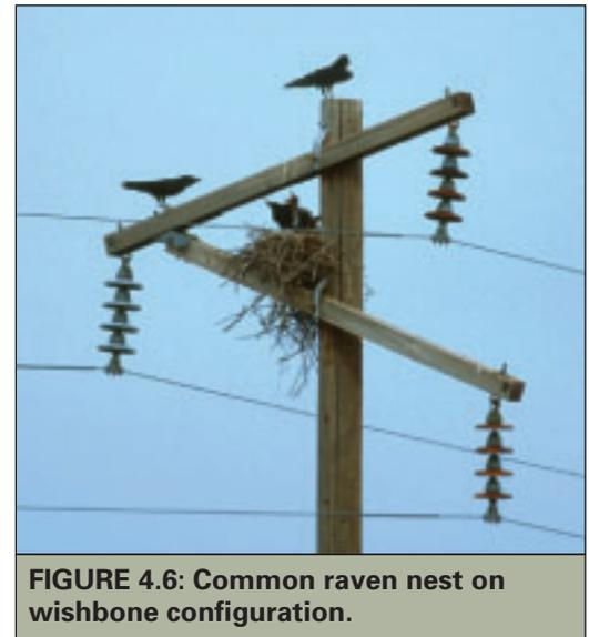
**FIGURE 4.6: Common raven nest on wishbone configuration.**
