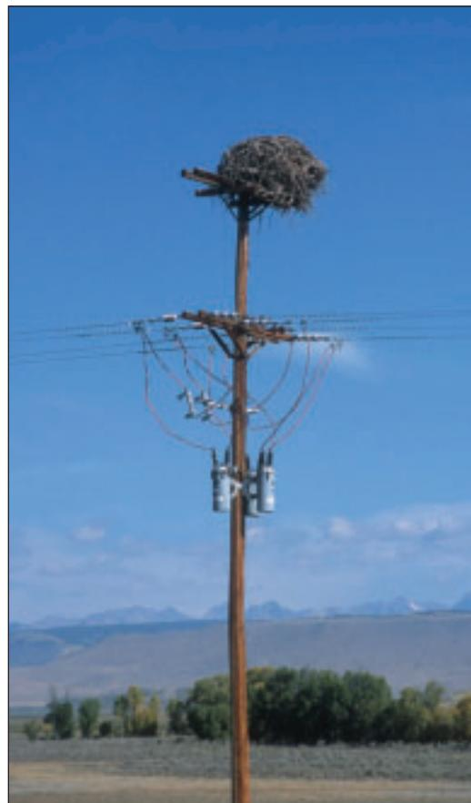
**FIGURE 6.16: Osprey nest in Wyoming atop double dead-end pole. Nesting material that may drop onto the conductors or equipment poses fire, outage, and equipment damage risks.**
