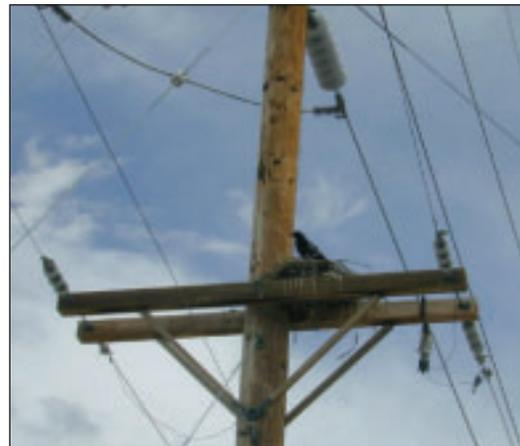
**FIGURE 6.6: Common raven nest on distribution underbuild of transmission structure.**
