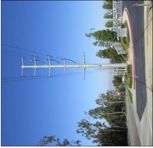
Typical 69kV Double-Circuit Steel Cable Pole with Only 1 Side Installed and 1 Side Pass Through
