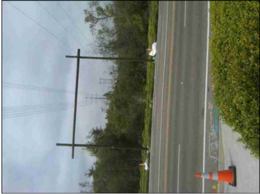
Typical H-Frame Guard Structure
