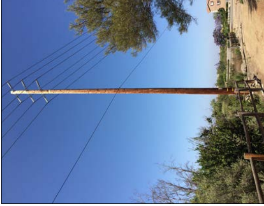
Typical 69kV Double-Circuit Tangent Wood Monopole
