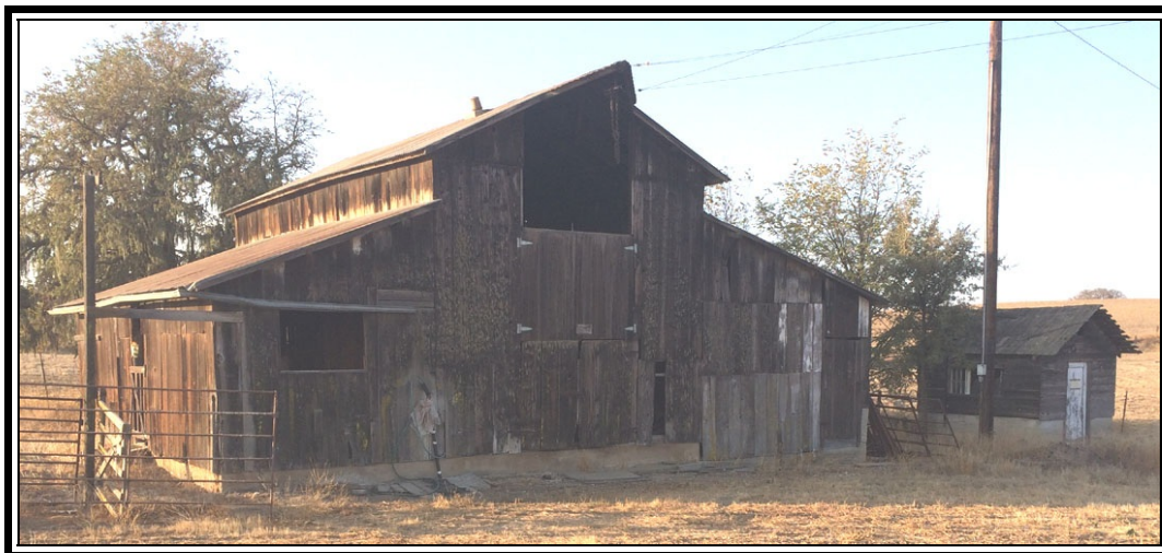
Monitor Barn-North Facade-Dimensions 40 Feet Across North Facade x 30 Feet Deep. Small Outbuilding To Right Dimensions ca. 8 feet On North Facade x 12 Feet Deep
