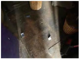
Photo 23. ACM: Floor tile mastic, partially covered with floor tile on View level.
