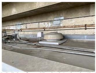
Photo 18. ACM: Rolled roofing on View level, Sections 2-40, above restrooms, concessions, and walkways.
