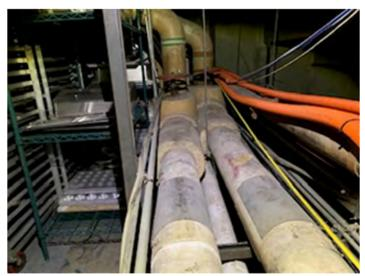
Photo 31. ACM: TSI fittings at hanger on foam straight run on Club level. Pipe chase is below seats. Foam insulation has an asbestos fitting every 10 feet; pipe also runs vertically from basement to View level.
