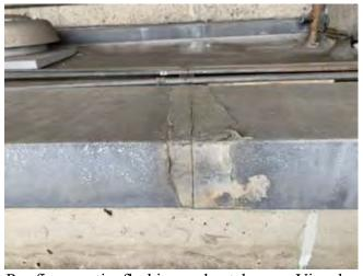
Photo 19. ACM: Roofing mastic, flashing and patches, on View level, Section 2-40.
