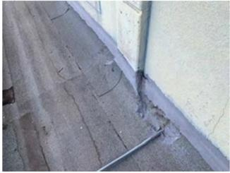
Photo 33. ACM: Roofing mastic at penetrations and patches on scoreboard building roof on Plaza level.
