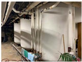
Photo 35. ACM: TSI tank insulation in HVAC room on level B2.
