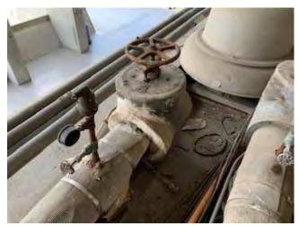
Photo 22. ACM: TSI elbows/fittings (large foam) on View level.
