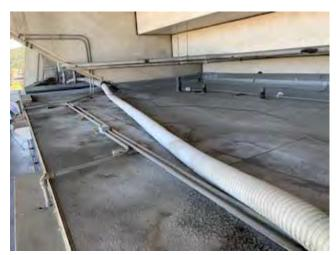
Photo 24. ACM: Roofing mastic at penetrations and patches, View level, section 41-49 and 54-61.
