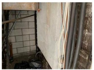
Photo 21. ACM: White stucco at fire hose boxes on View level.
