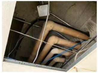
Photo 26. ACM: TSI elbows in pipe chase between restrooms and above ceilings, Press level.
