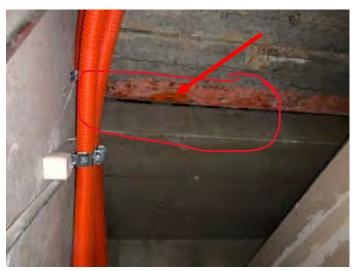
Photo 30. ACM: Mastic under seats between concrete slab and I-beam, sections 1 – 40, Club level.
