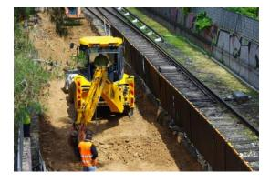
A construction barrier is built at the edge of the site to protect tracks from adjacent work.
