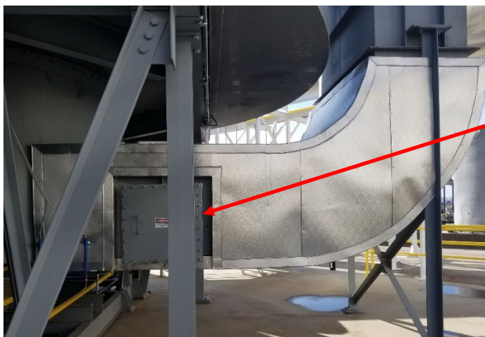
Figure OMP-1A RTO Odor Sample Port Location
