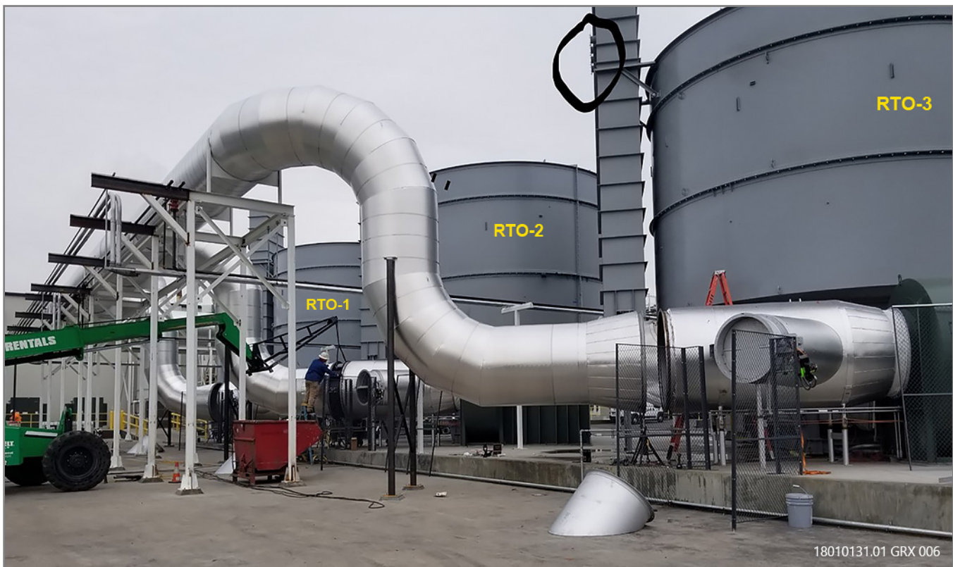
Figure 2-7 Newly Installed (as of December 2018) RTO Inlet Connections at Diamond's Ripon Facility
